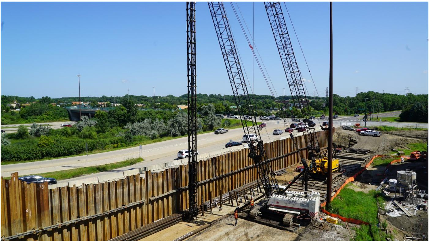
Crews are installing sheet pile and associated infrastructure to support the future LRT tracks. Significant amount of sheeting for the SouthWest Station has been completed. Crews will transition to working on the bridge structure crossing Technology Drive and Prairie Center Drive.
