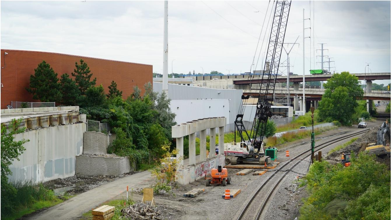
The old Glenwood bridge is almost fully demolished. Crews removed the deck and girders that once spanned the rail corridor and bike trail. Work on retaining walls, bridge abutments and piers continues in the area. Work activities are coordinated with active freight traffic.
