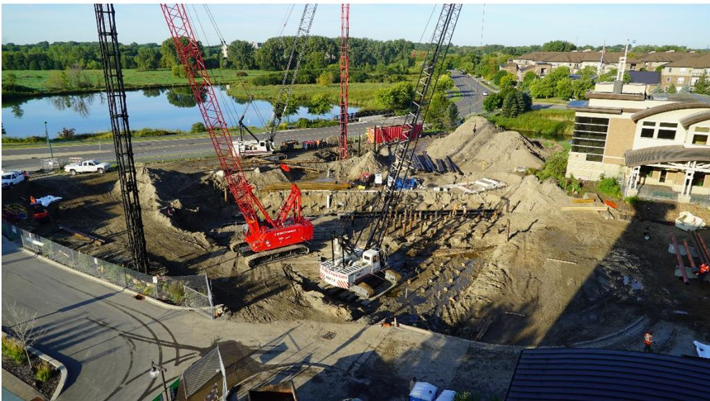
Crews install piles that will be part of the future SouthWest Station area. Coming this Fall, crews will construct a temporary passenger waiting area for bus riders and demolish the current SouthWest Transit Station passenger waiting area and former offices. Work will then progress on building the shared bus and LRT facility.
