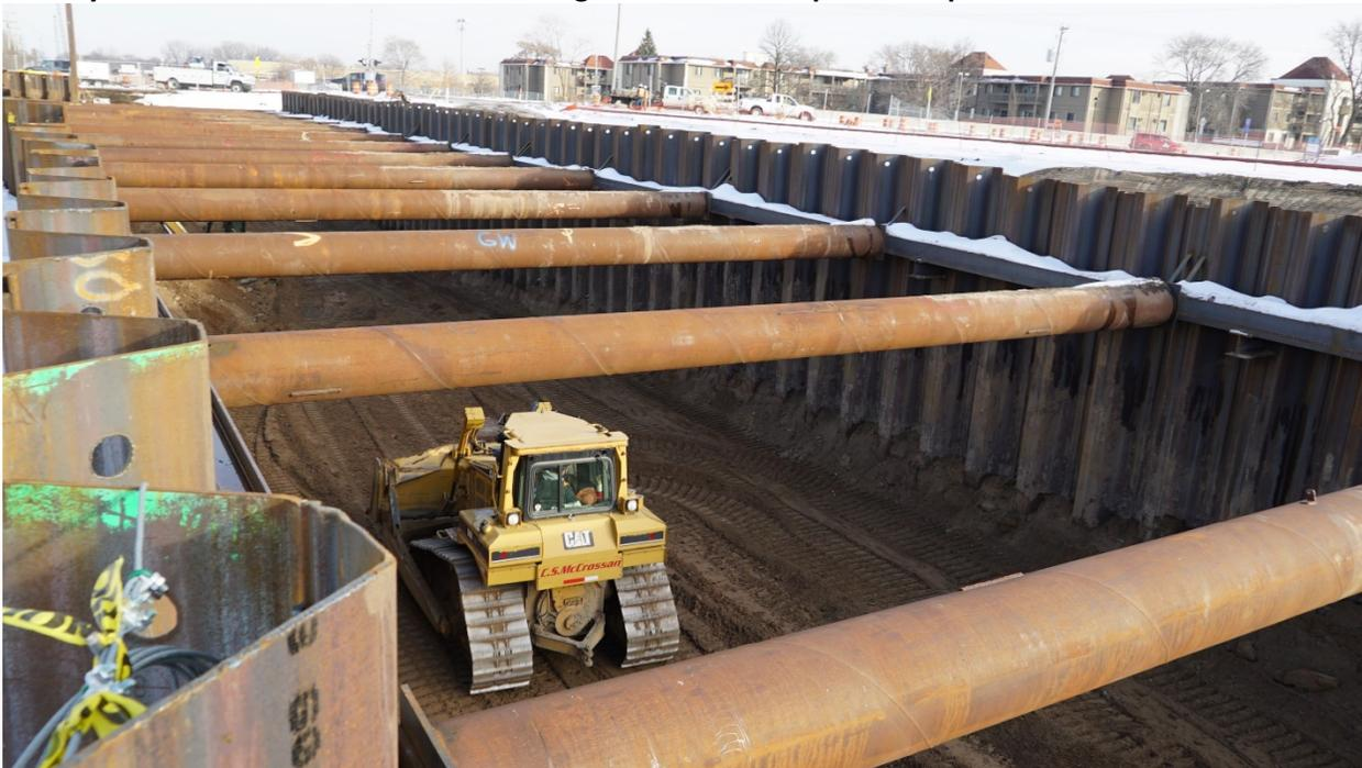
Excavating and grading work for the South Cedar Lake Trail underpass continues at Blake Road in Hopkins. When complete, the new underpass will enable trail users to cross under Blake Road instead of interacting with vehicle traffic, improving pedestrian and bike safety in the area.
