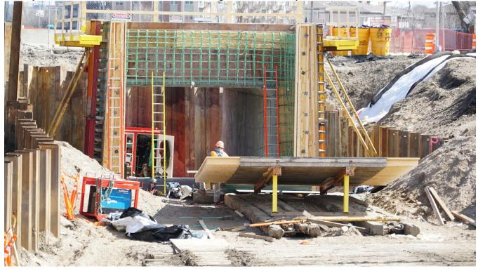
Workers construct the box structure on the approach to what will become the Wooddale underpass. Crews have been conducting piling and excavation work. The work has progressed to a point where we are ready to begin the full closure of Wooddale Avenue on Thursday, April 23 and continue with these activities into the roadway.
