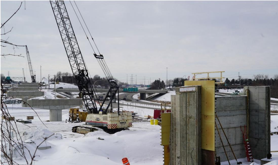
Crews have progressed the piers and abutments for the new LRT Bridge along Valley View Road, which includes piling and concrete work. Soon bridge girders will be put in place.
