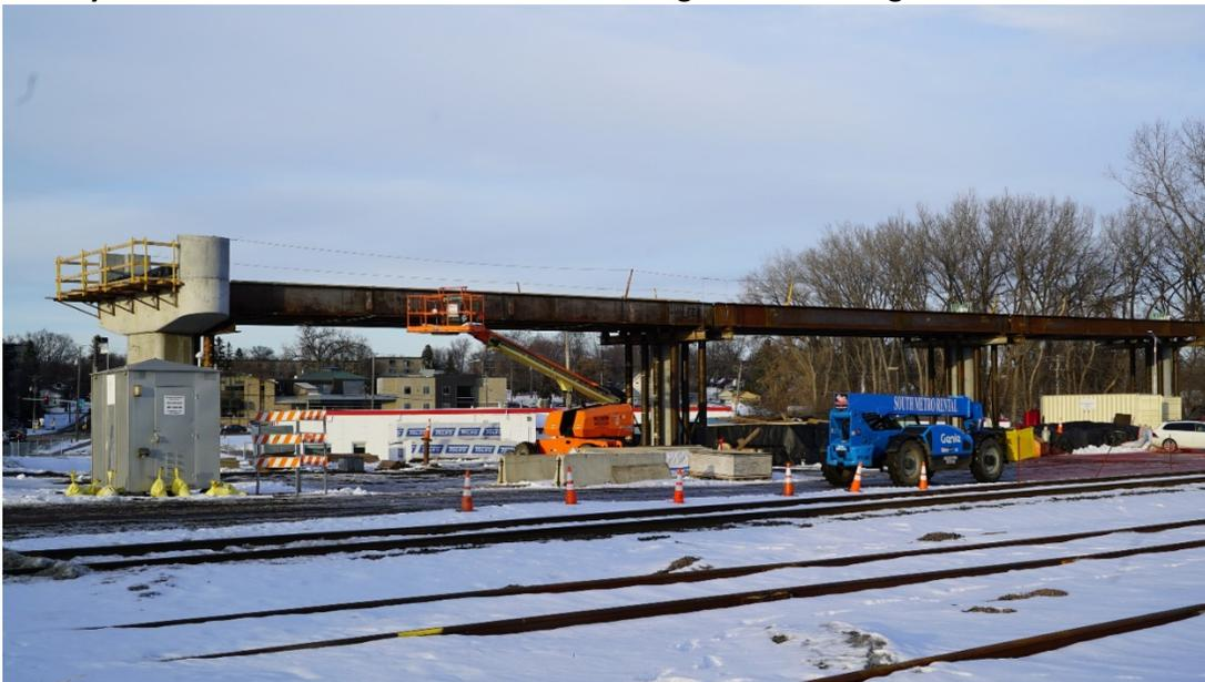
With much of the pier work complete, spans are being set for the Beltline Boulevard Regional Trail Bridge. Crews will be working to set rebar and “falsework,” items that are used just for construction, to advance bridge spans and deck. Once completed, regional trail users can use this safer route to cross Beltline Boulevard and continue on the South Cedar Lake Trail.
