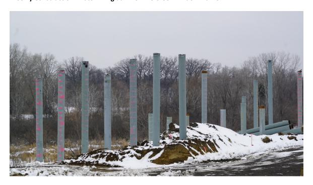
Work to install piles to support LRT infrastructure is ongoing in the area. Piles are driven into the ground until they reach the proper depth and then are cut-off to the appropriate height.
