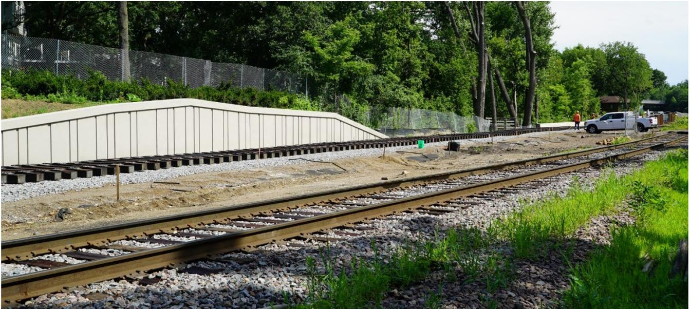
Construction of the new, permanent freight rail alignment on the approaches to the Cedar Lake Channel is almost complete. Ballast and freight rail ties have been installed and freight rail track is starting to be pulled through the area. Freight rail will shift onto this newly construction track, potentially next week on Wednesday July 22, pending coordination with the freight railroad.
