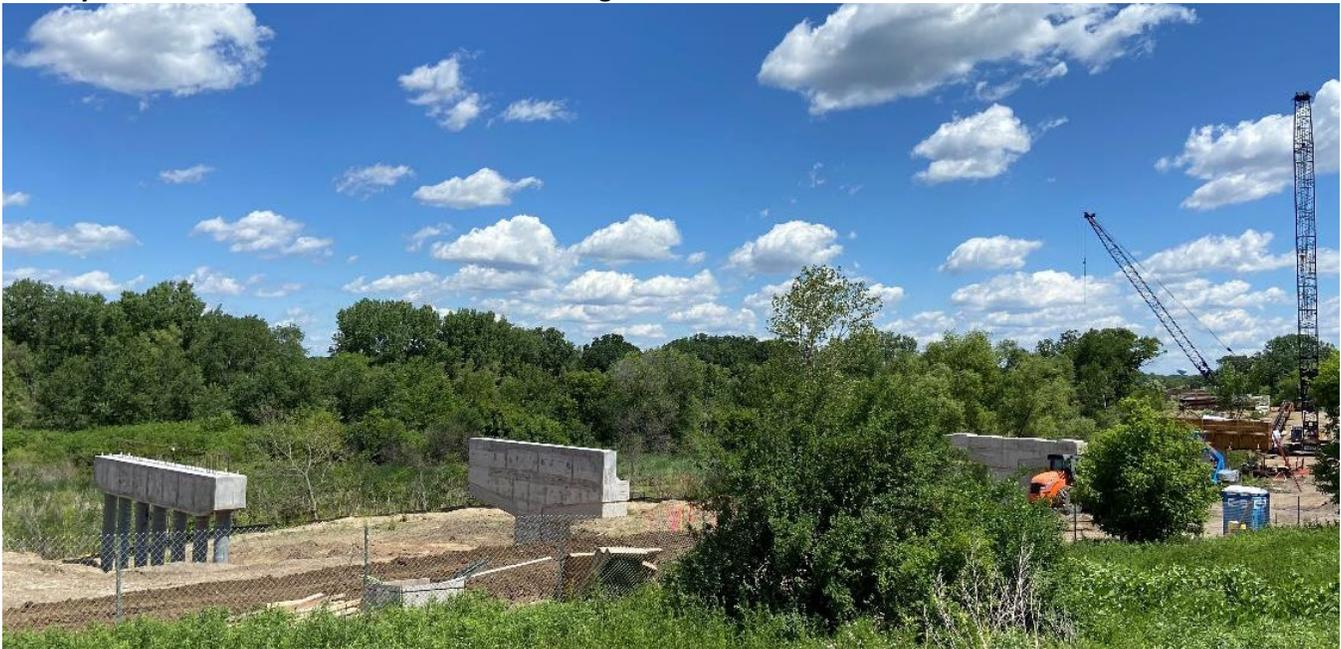
Many of the piers for the Nine Mile Creek bridge are nearing completion. Both piling and concrete work continue in the area as crews construct bridge foundations.
