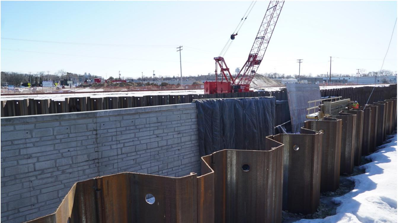
Crews are building the walls for the regional trail underpass at Blake Road. This photo shows the wall texture a trail user will see as they pass through the tunnel. The tarps are used to help keep the concrete warm, as it cures in colder temperatures.
