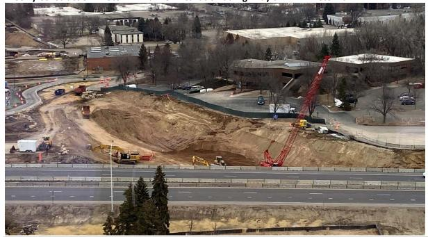
Crews continue excavation for the LRT tunnel under Highway 62, with concrete work creating the base slab of the north tunnel portal.
