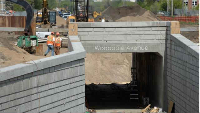
When the South Cedar Lake Trail reopens, bikers and pedestrians will be able safety travel under vehicle traffic to cross Wooddale Avenue. The underpass has clearly taken shape and crews are completing the tunnel form, and then will reconstruct Wooddale Avenue. The roadway is anticipated to open to traffic by early June.
