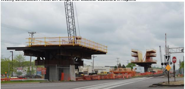
With the LRT bridge piers nearing completion, the structural forms to take the bridge over the roadway and freight rail are starting to take shape. The form work in the front image is called a pier table, which taken quiet literally means the base or "table" for the bridge to be placed on the piers. The bridge structure is a post-tensioning box girder. This type of bridge can efficiently span long distances. The initial shape of the box girder is visible on the second pier in the background.
