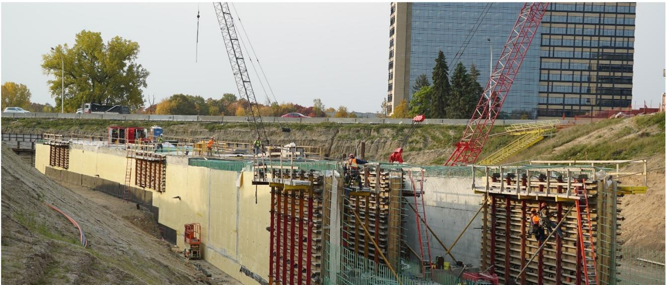
Notable progress has been made on the LRT tunnel's eastern segment under Highway 62. Tunnel walls and roof continue to take shape. The tunnel structure in this photo will be all underground when complete.
