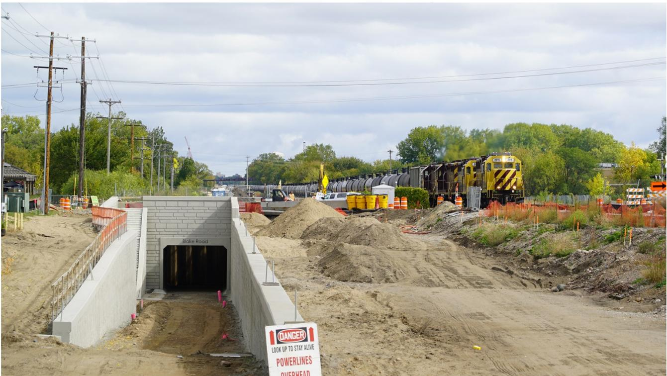
Crews have almost completed the western portion of the regional trail underpass at Blake Road, allowing them to remove the excavation supports. Work on the tunnel will continue into next year.
