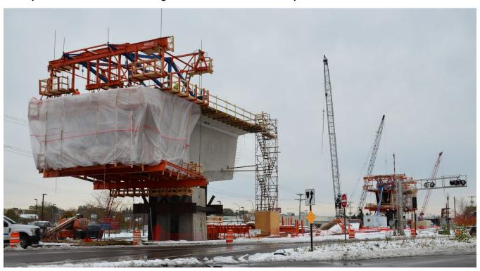
The LRT bridge spans continue to take shape at Excelsior Boulevard in Hopkins. To construct the bridge, crews are using a system called a form-traveler to build the spans between the piers. Instead of setting beams, the bridge structure is formed a section at a time. The bridge structure is called a post-tensioned box girder bridge,
