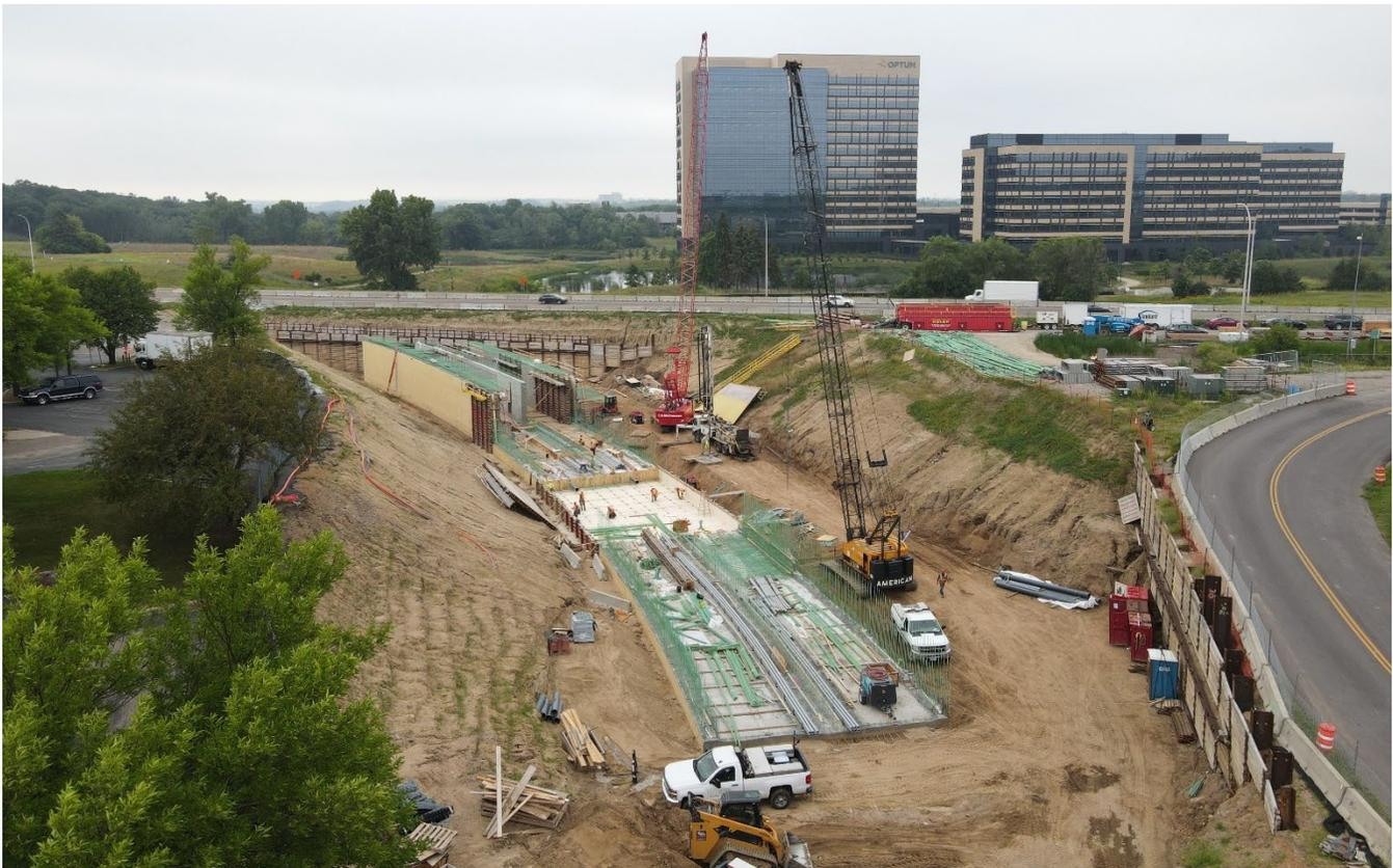
The construction of the LRT tunnel under Highway 62 is a multi-year process. With traffic shifted onto one side of the Highway crews have built the base of the tunnel and are working to progress walls and roofing.
