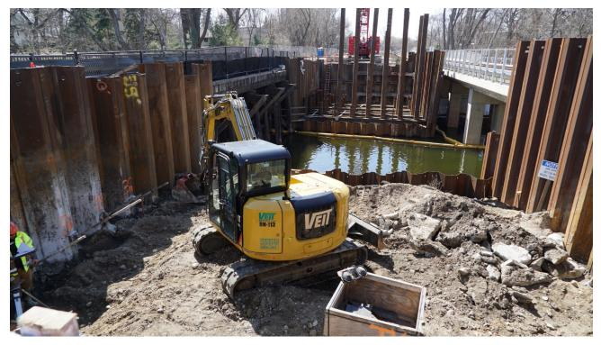
Crews have been working to excavate the abutment for the north end of the Cedar Lake Channel LRT bridge. Piling for this abutment has begun. Piles can be seen in the photo for the south abutment. The new freight bridge is also pictured on the right.
