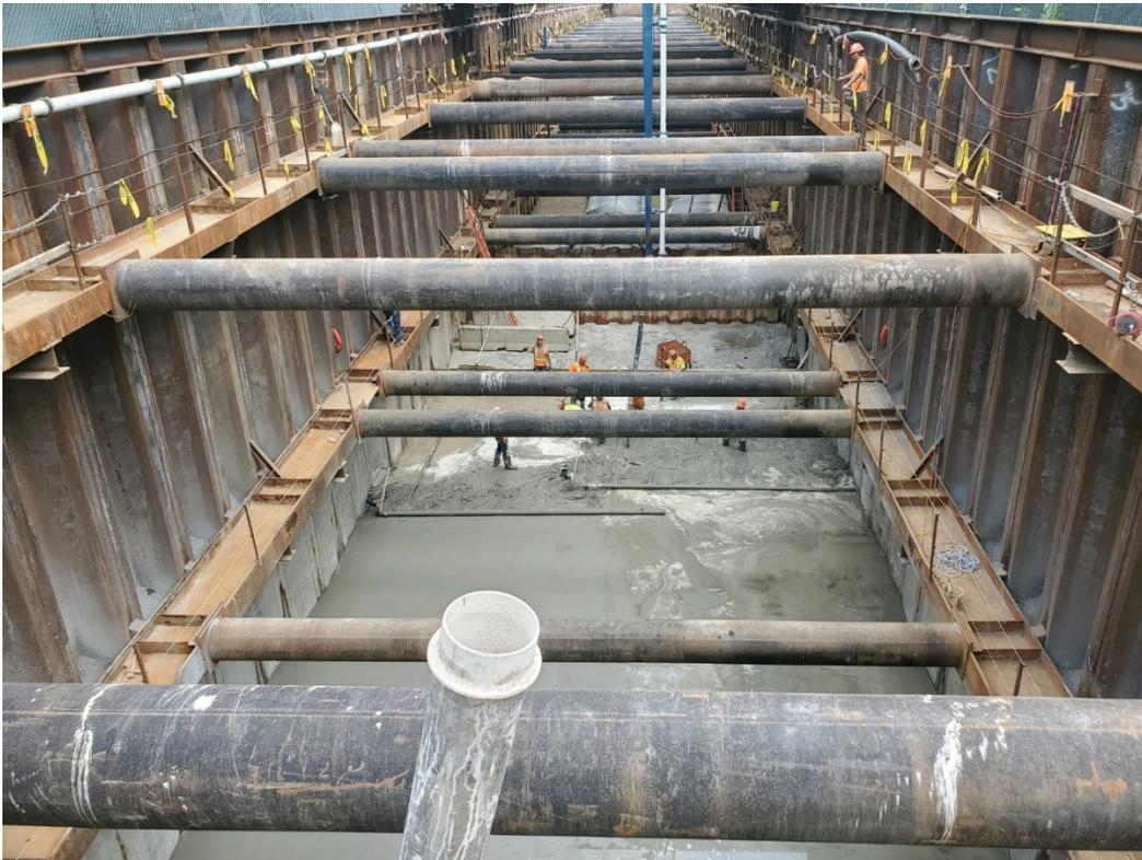
A view into the Kenilworth Tunnel as crews work on concrete at the base of the tunnel, called a leveling slab. Crews work cell by cell, excavating, installing lateral supports, and pouring concrete. There will be a waterproof membrane around the concrete tunnel structure.
