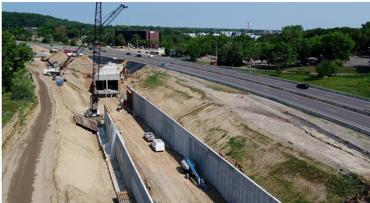
A view looking north of the LRT tunnel that passes under Highway 62. Retaining walls are currently under construction connecting the tunnel portal.
