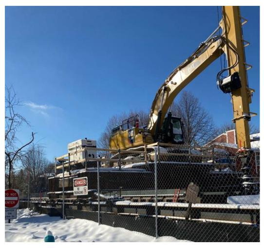
To excavate deep into the tunnel cell, crews use equipment called a telledipper excavator (pictured). Crews are working to fully excavate the first tunnel cell in February. Crews were not able to work over the past week due to the extreme cold.
