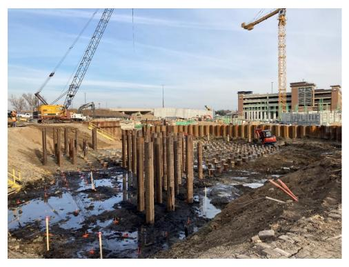
Looking east towards SouthWest Station construction crews install piles that will support the bus loop/roadway. Due to poor soils conditions, project elements including track, stations, roadway and utilities are supported by piles.
