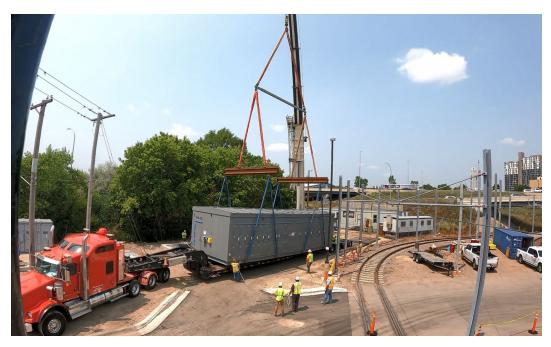
Crews place the TPSS into position, which had been fabricated off site. As the day progresses you can see crews plan, inspect, and install the TPSS.
