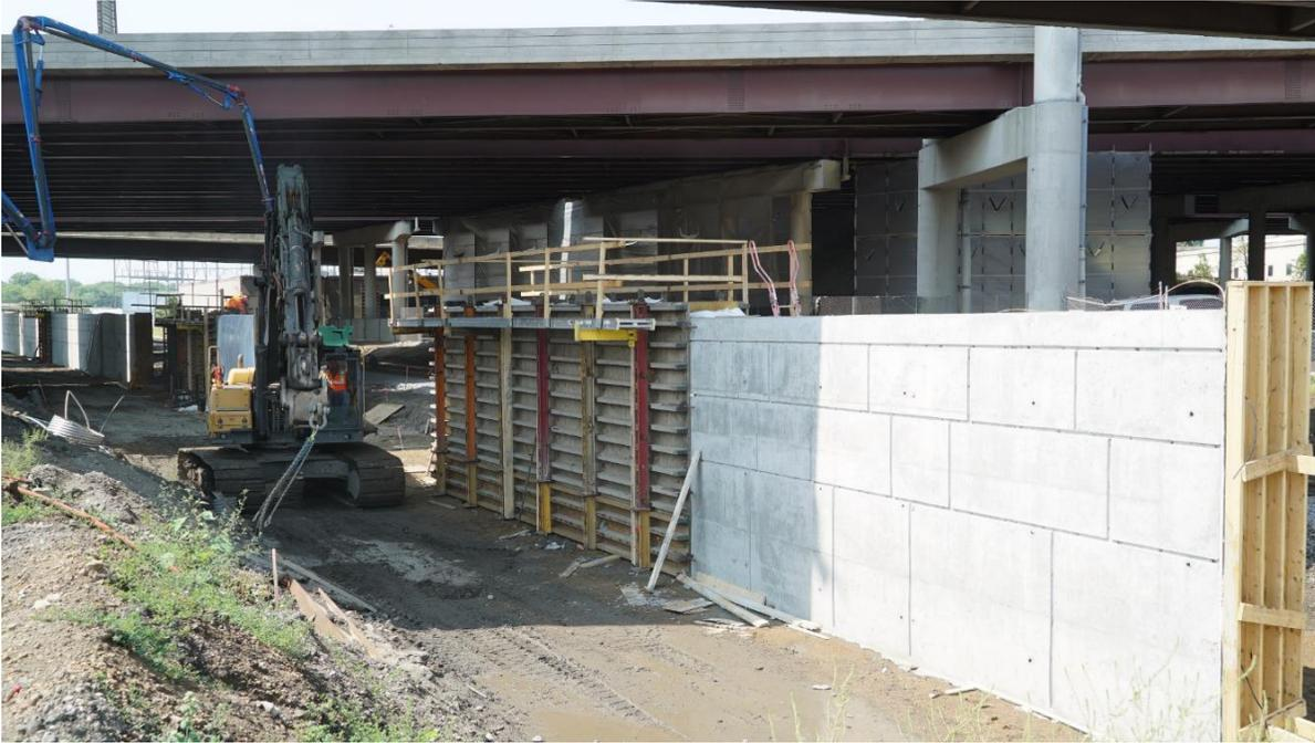
Crews are building sections of the corridor protection wall between the existing BNSF freight rail mainline tracks and the Southwest LRT tracks under construction. The concrete is complete in the foreground of the photo. In the background, formwork is complete and ready for crews to pour concrete.
