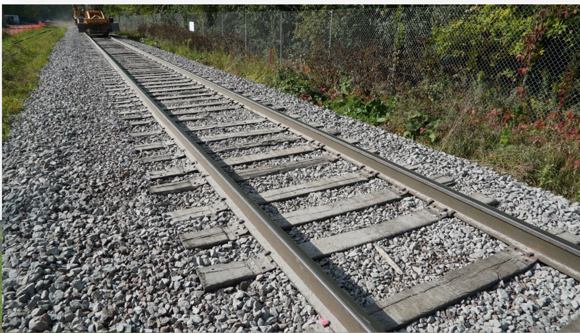
New Freight Rail Track
