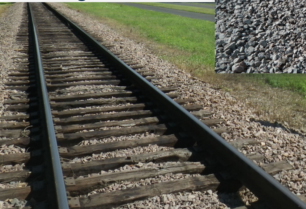
Old Freight Rail Track
