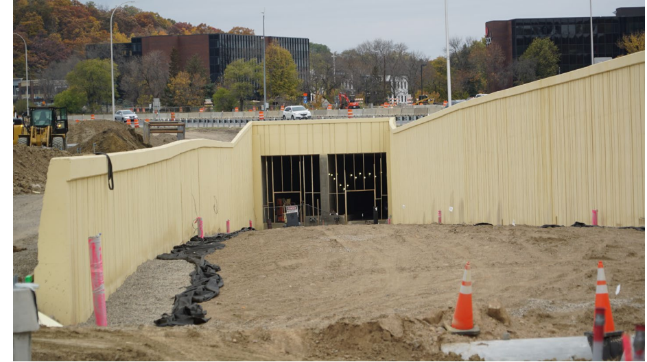
Highway 62 LRT Tunnel
