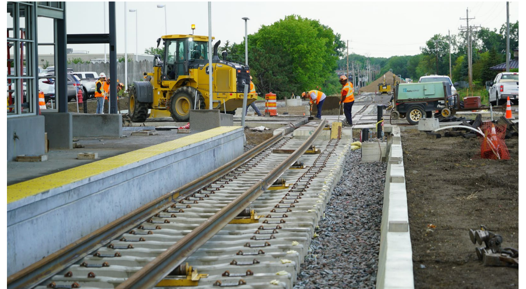
LRT track at the Downtown Hopkins Station
