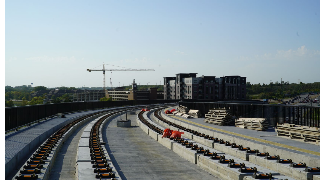
Prairie Center Drive LRT Bridge
