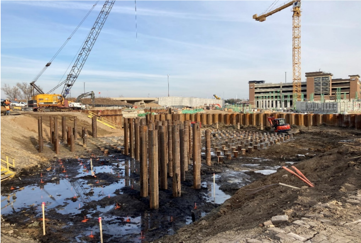
Looking east: pile supports for bus loop
