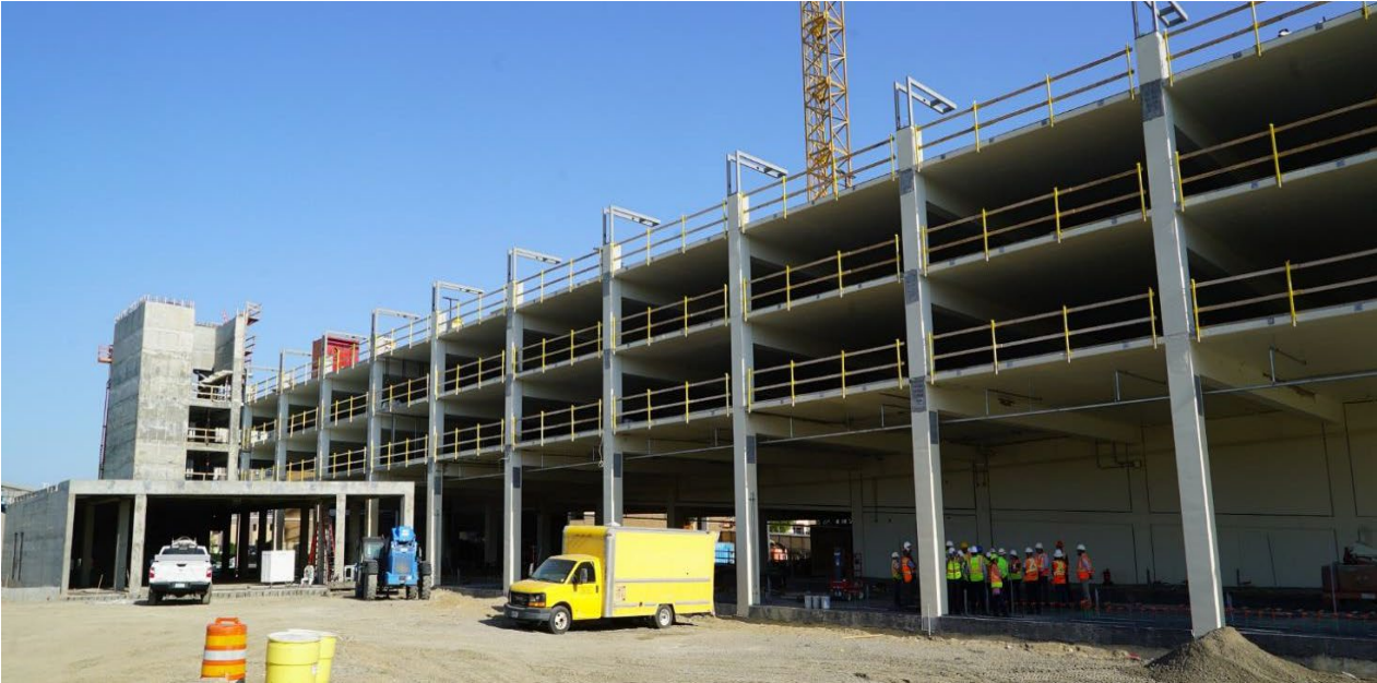
Looking east: construction of the parking ramp, station & waiting area
