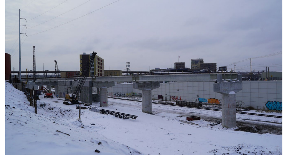
Glenwood Avenue Bridge
