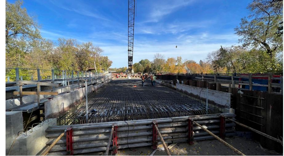
Cedar Lake Channel LRT bridge to be completed this year
