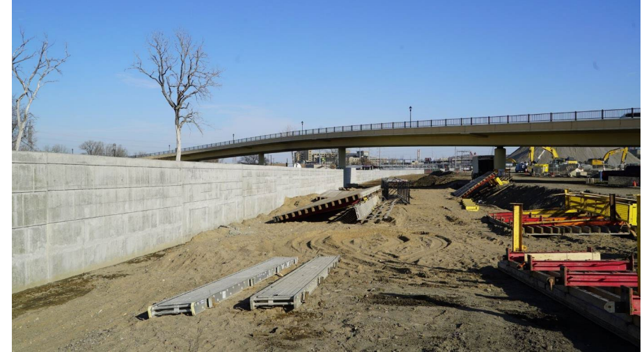
Corridor Protection Wall
