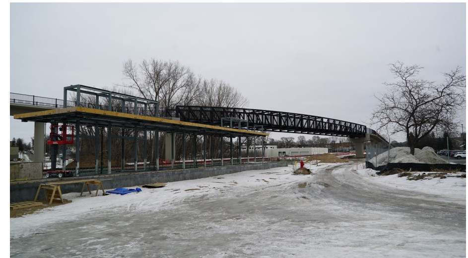
Beltline Boulevard Station
