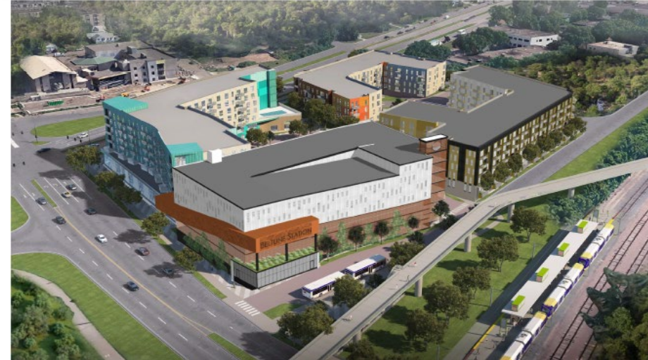
Beltline Station Development, St. Louis Park
