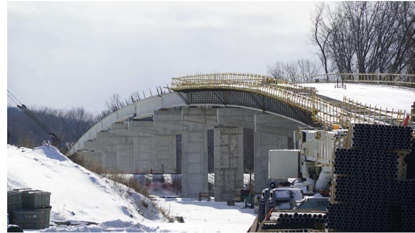
Minnetonka-Hopkins LRT Bridge
