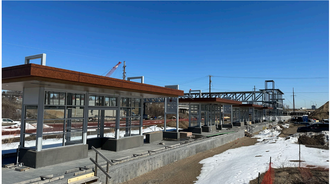
Photo of the Bryn Mawr LRT Station area under construction, April 2023
