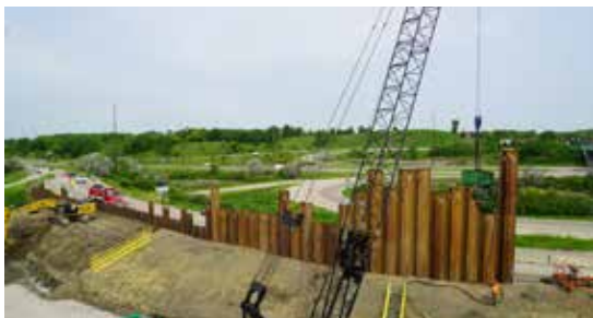
Pile driving near Southwest Station in Eden Prairie
