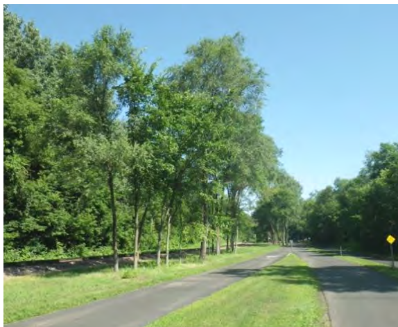
a. View looking north of the Burnham Road Bridge
