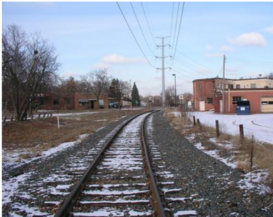
Figure #2- Locomotive Engineer's viewpoint when approaching the Walker Street crossing from the North. This is the same distance and opposite direction as from Library Lane from the North. 243 ft. of visibility.
