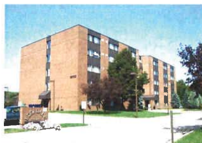
Edendale Housing Improvements
