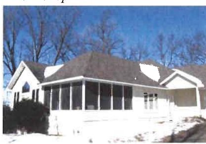
Senior Group Home, Rehab Project
