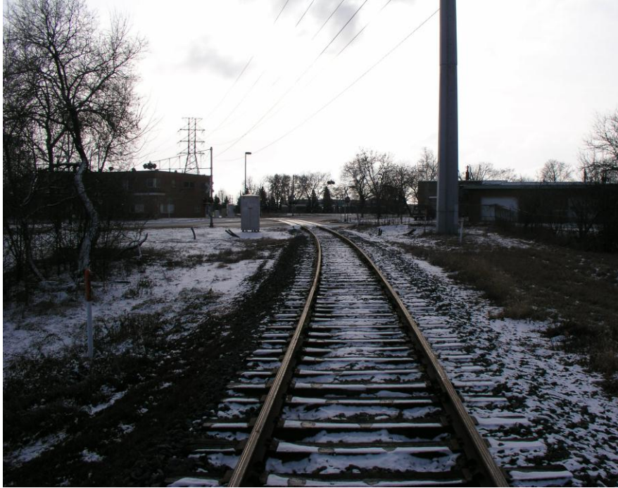
Figure #3 - Locomotive Engineer's viewpoint when approaching the Library Lane Crossing from the North. Only 178 ft. of visibility.
