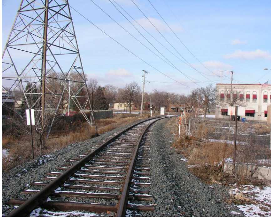
Figure #1- Locomotive Engineer's viewpoint when approaching the Walker Street crossing from the South. 247 ft. of visibility.
