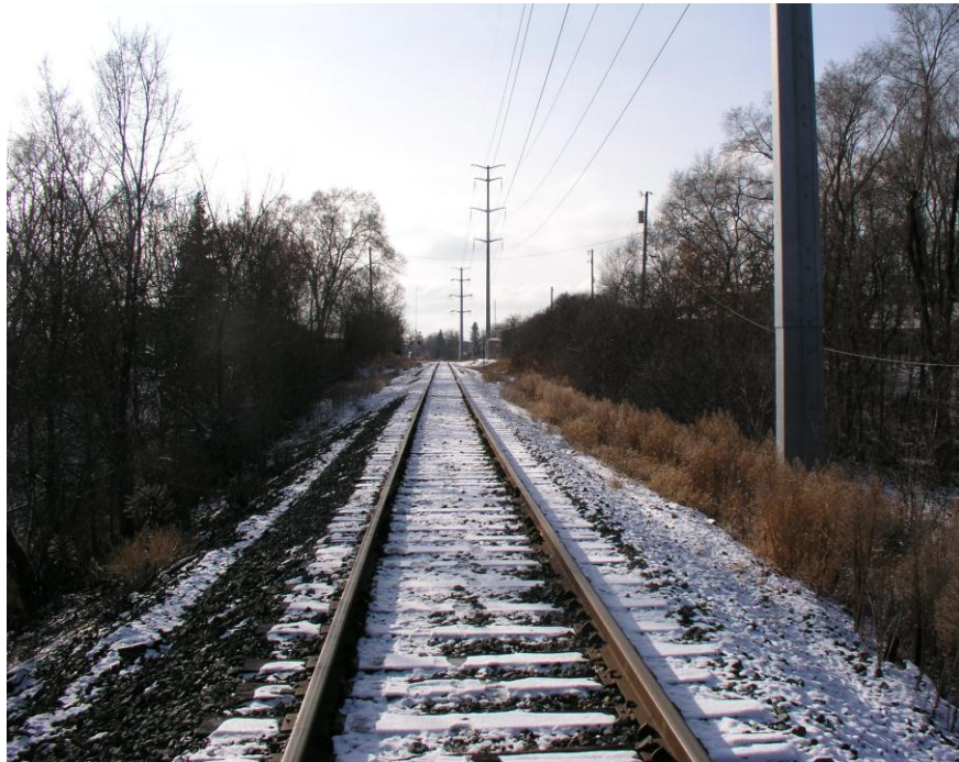
Figure #6- Locomotive Engineer's viewpoint when approaching the Dakota Ave. crossing from the North. 479 ft. Very little visibility except straight ahead.
