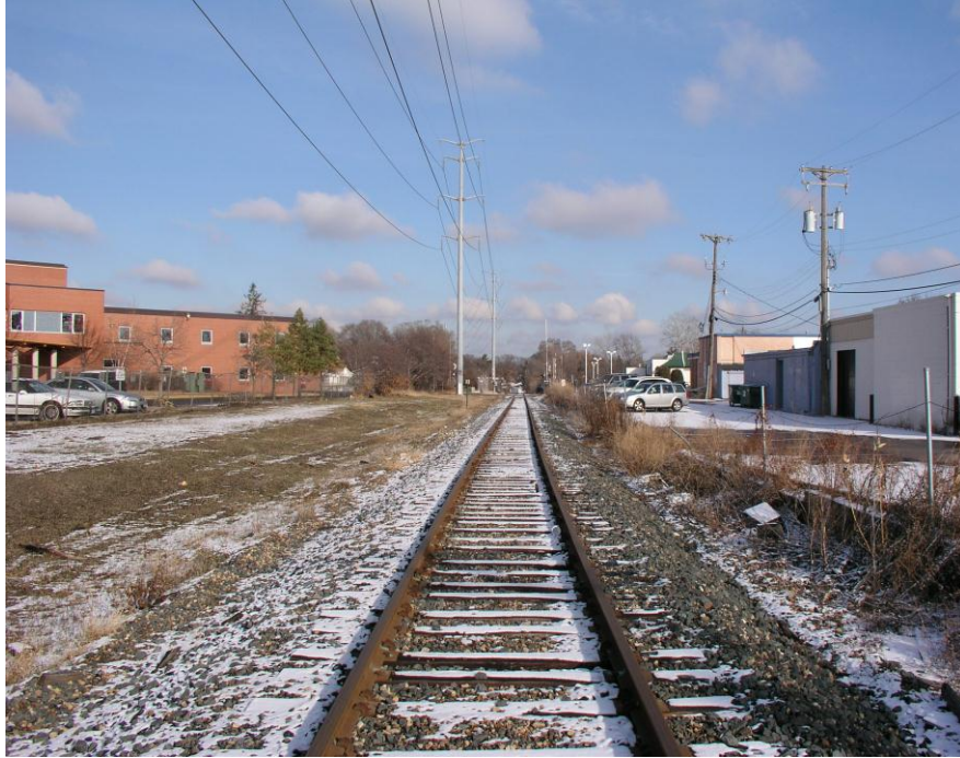
Figure #5 - Locomotive Engineer's viewpoint when approaching the Dakota Ave. Crossing from the South. 434 ft. of visibility.
