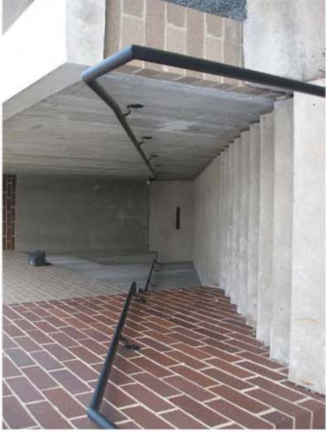
LOOKING EAST (SOUTHWEST CORNER OF THE BUILDING)
