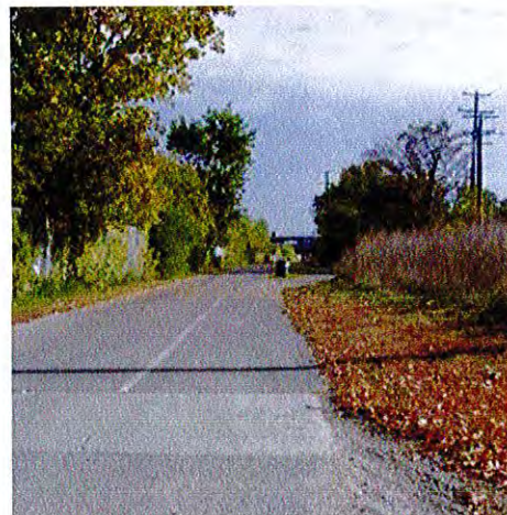
From Linden Avenue junction, looking northeast along Cedar Lake Regional Trail
