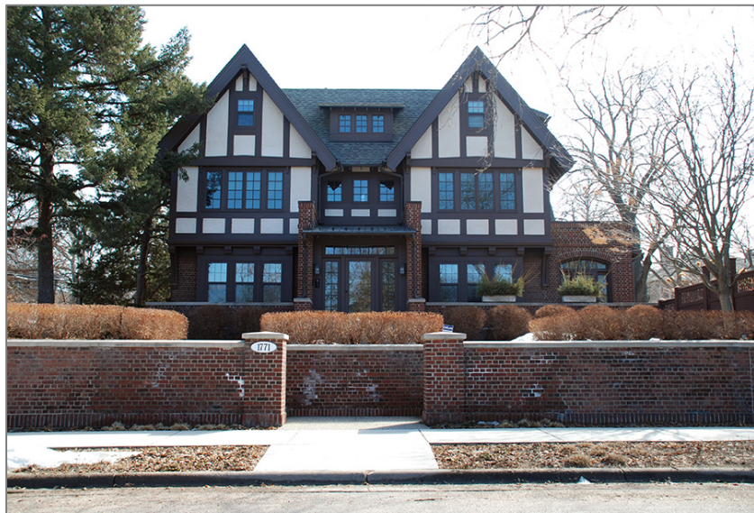
Figure 5. 1771 Logan Avenue South, Facing East
