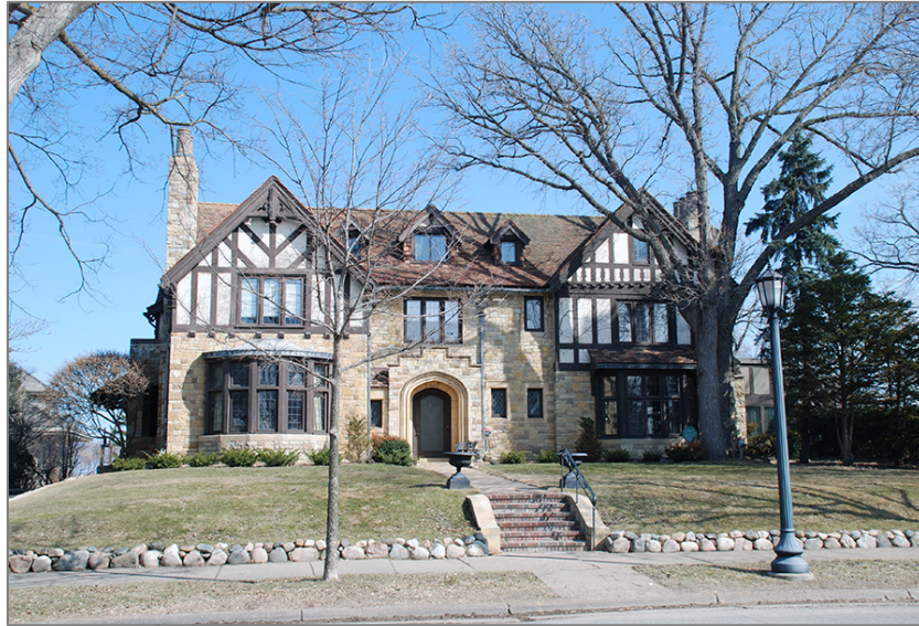
Figure 6. 1314 Mt. Curve Avenue, Facing North
