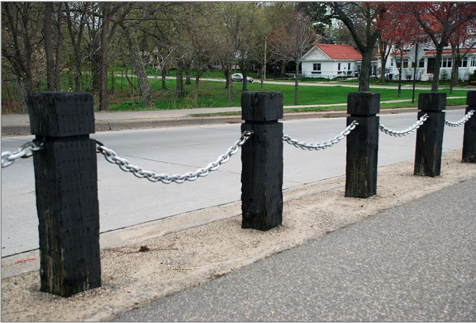
Figure 80. Guardrail along West Lake of the Isles Parkway, facing southwest
