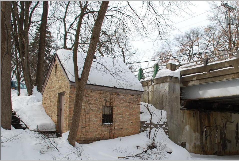
Figure 61. Pump House, facing southwest
