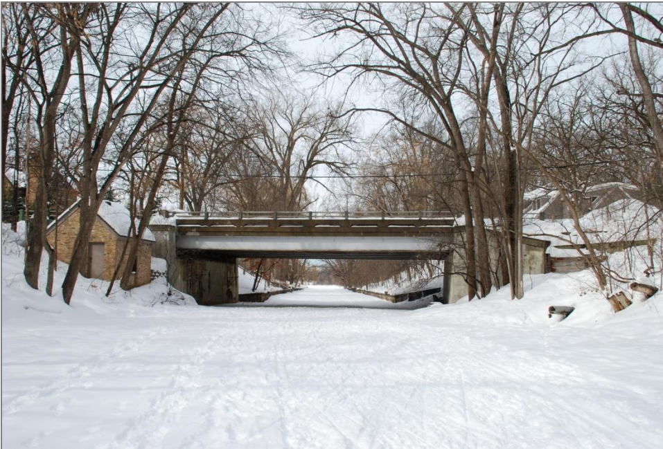
Figure 65. Bridge No. 6, facing northwest
