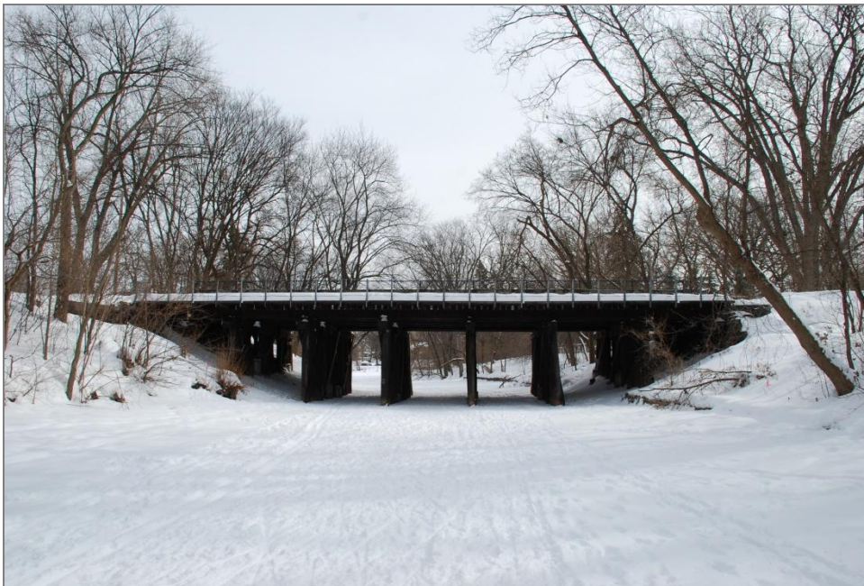
Figure 63. Bridge No. 5 (M&StL, now TW&C), facing southeast
