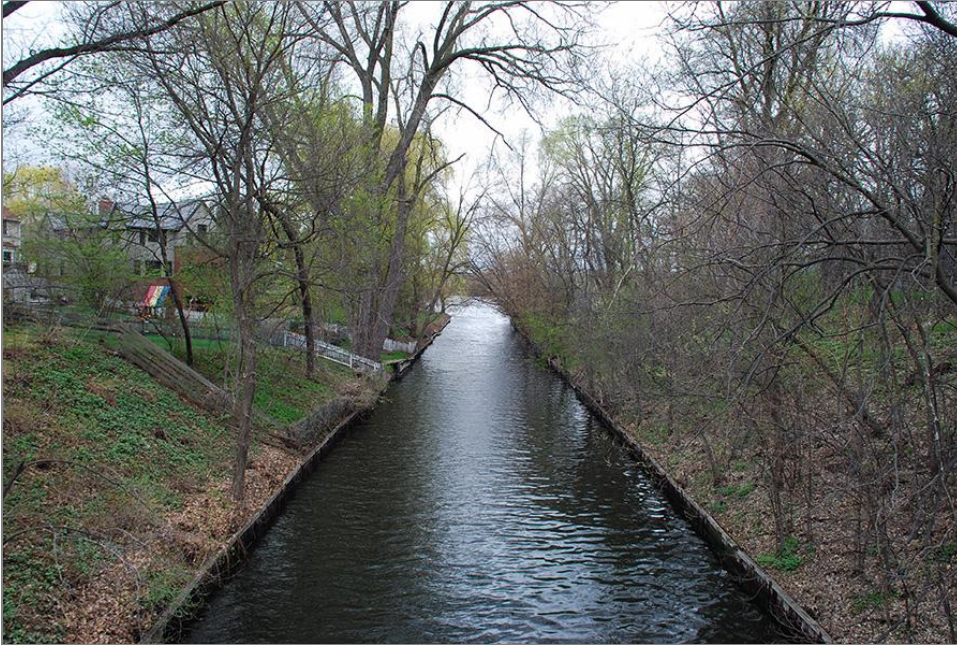
Figure 45. Channel, facing northwest from Bridge No. 6
