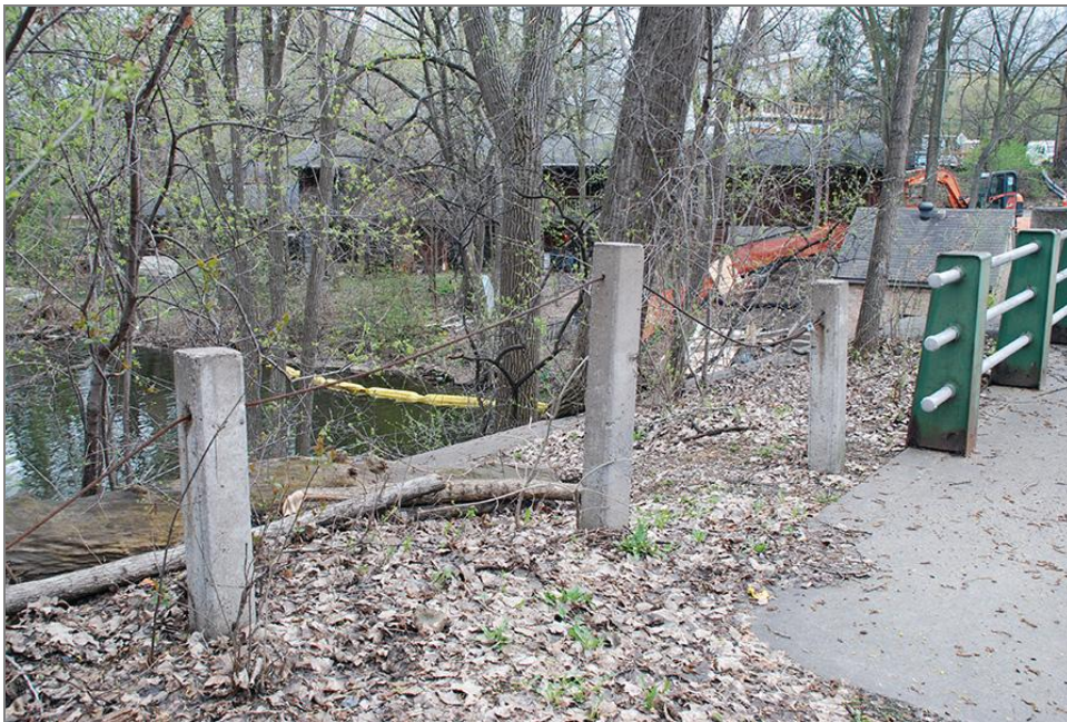
Figure 82. Guardrail on the east side of Burnham Road, north of Bridge No. 6, facing southeast
