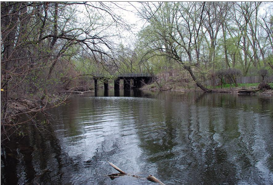
Figure 41. Area between the bridges, with Bridge No. 5 in the distance, facing southeast
