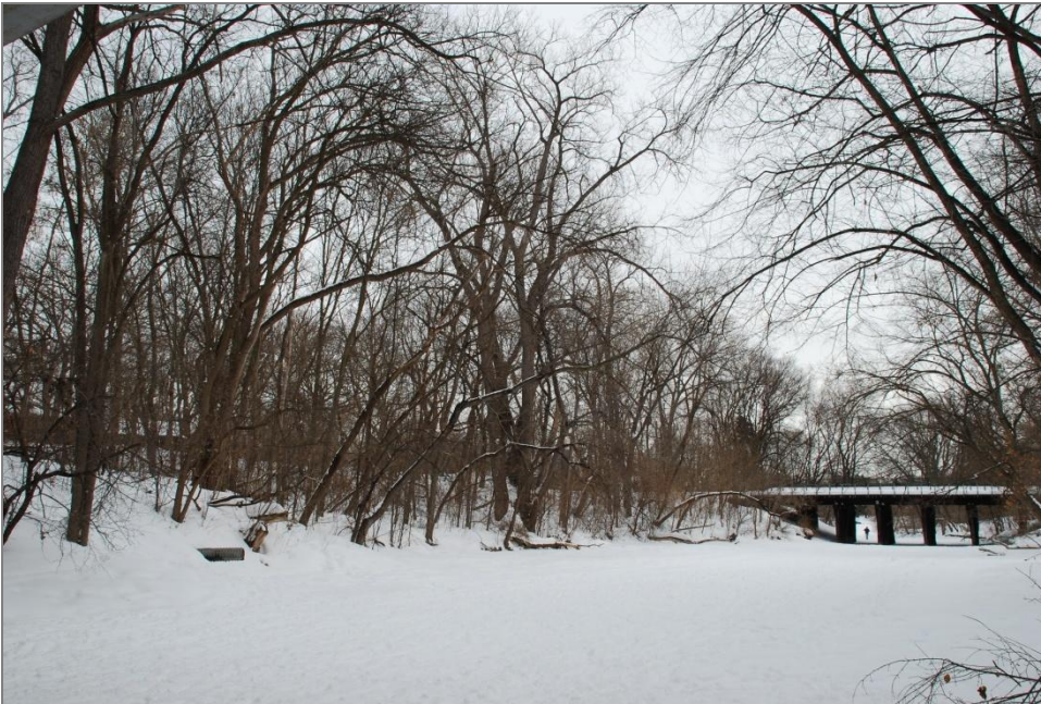
Figure 40. Area between the bridges, with Bridge No. 5 in the distance, facing east
