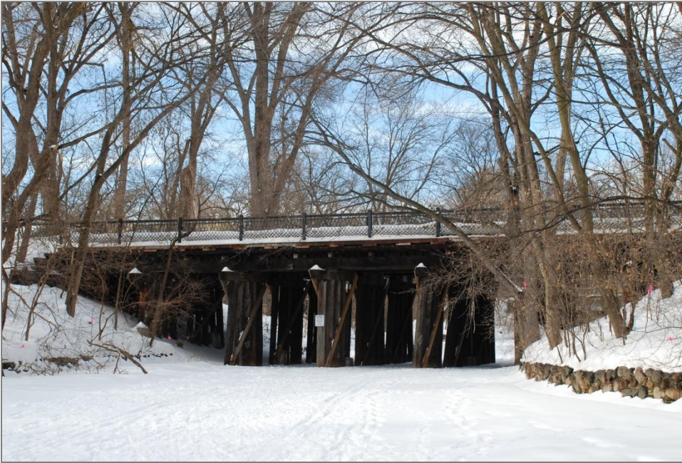
Figure 64. Bridge No. 5 (Bridge 27A43, M&StL, now Kenilworth Trail), facing west
