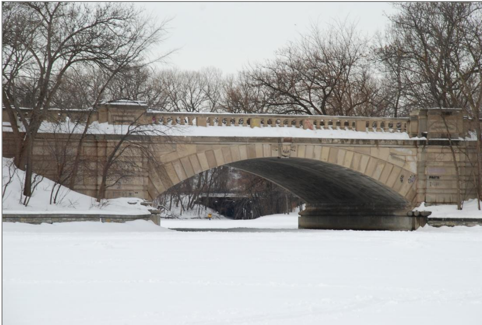
Figure 62. Bridge No. 4, facing northwest
