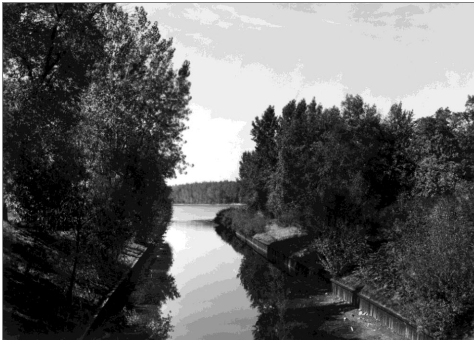
Figure 20. Sheet piling installed by WPA along Kenilworth Lagoon near Cedar Lake Avenue, 1936 (Minnesota Historical Society Collection)
