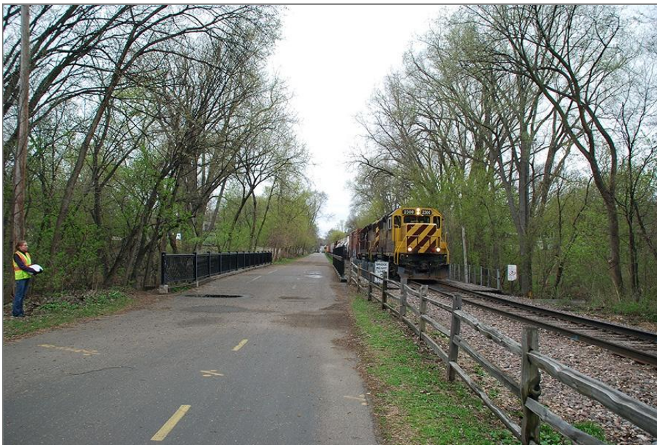
Figure 55. Kenilworth Trail and the M&StL/TC&W railroad line passing over Bridge No. 5, facing southwest
