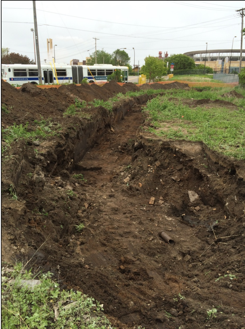
Figure 8. Photograph of trench looking east.
