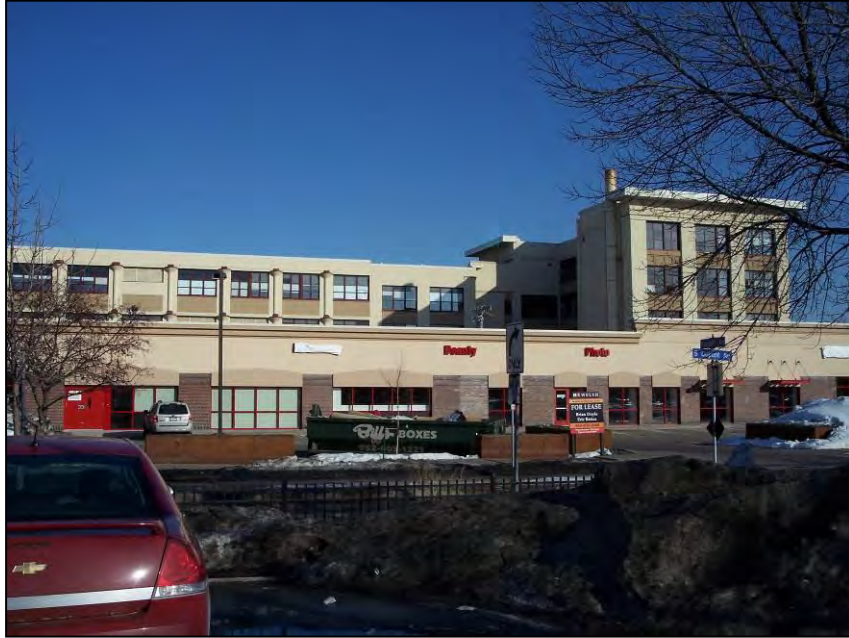
Above: West facade (modern building in foreground). View to east.
