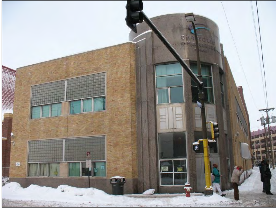
Warner Brothers Picture Distribution Building, 1000 Currie
