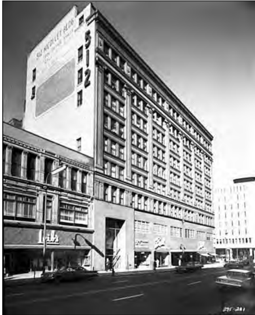
512 Nicollet Building (formerly the Andrus Building), 1965 Norton and Peel, photographer—Minnesota Historical Society Collections
