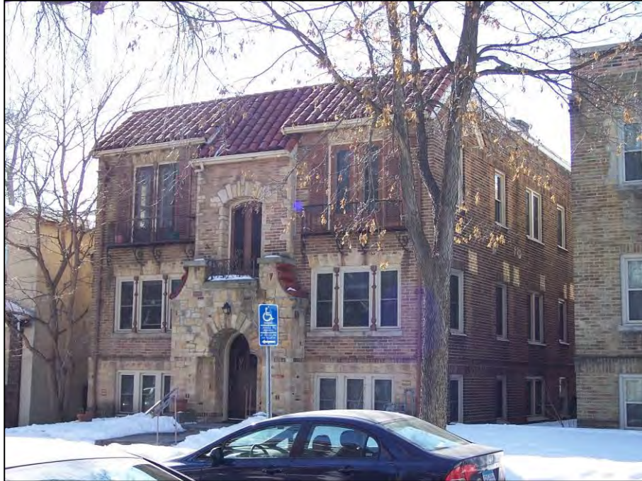
The M. E. Greenberg Building, 2884 Irving Avenue South
