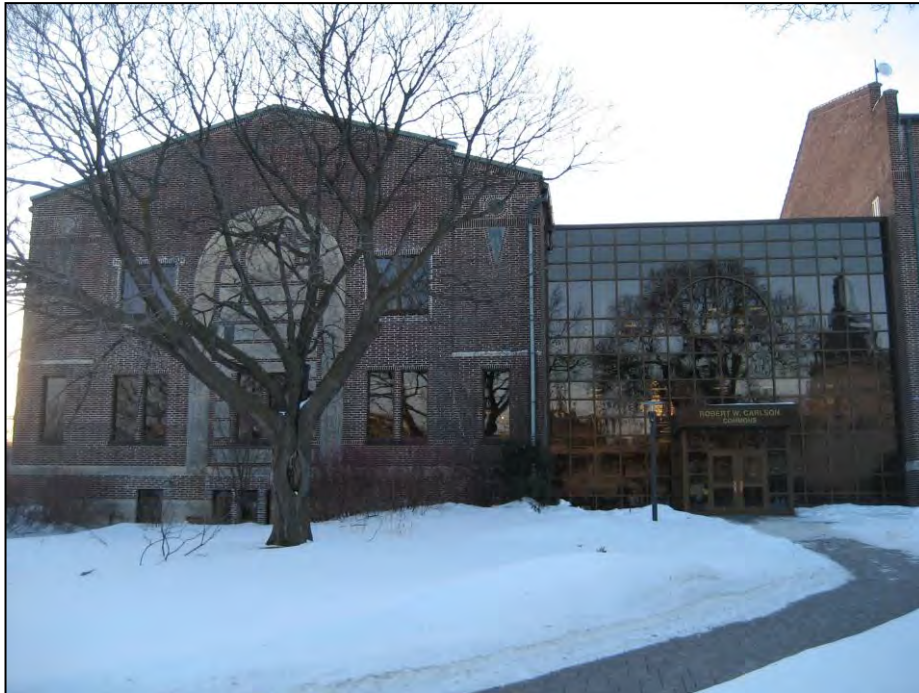
Above: Front facade, looking northeast
