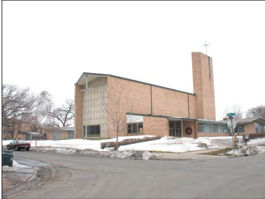
Above: Sanctuary and entry at corner of Stevens Avenue and Twenty-second Street. View to southwest.
