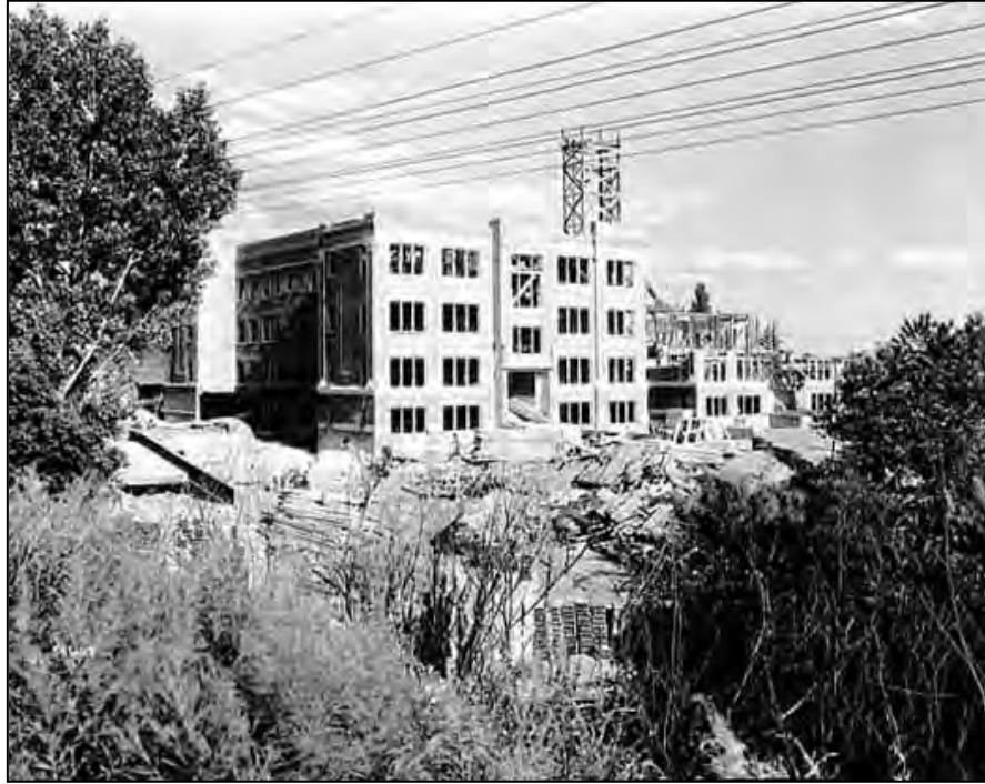
Calhoun Beach Apartments under construction, 1925 Hibbard Studio photograph—Minnesota Historical Society Collections
