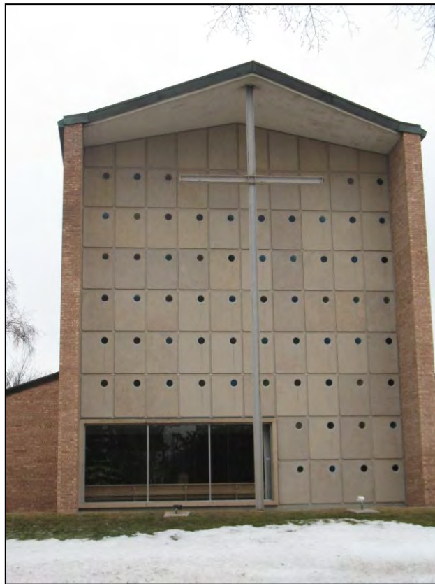
Below: Detail of east facade.
