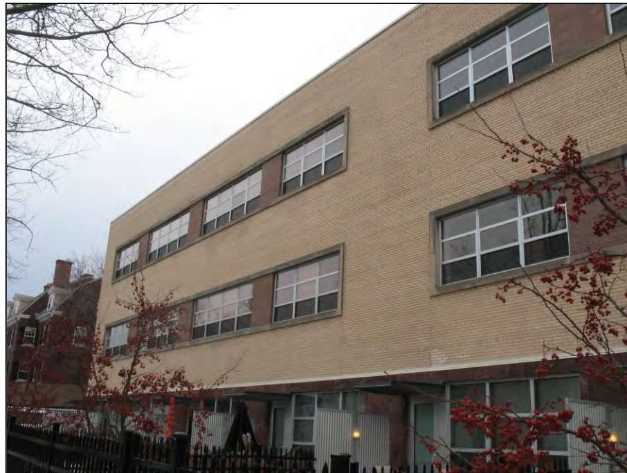
Looking southwest at the Stevens Avenue (east) facade where the basement was modified to accommodate apartment units.
