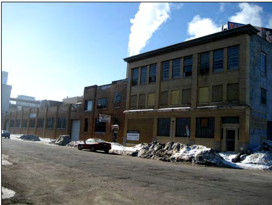
Top: Front facade of 1909 section, with Seventh Avenue side to right.
