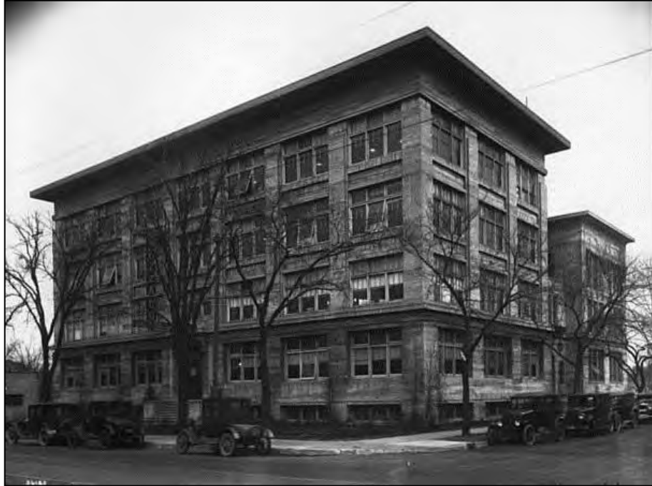
Lake Street facade, c. 1920. Charles J. Hibbard, photographer—Minneapolis Historical Society Collections
