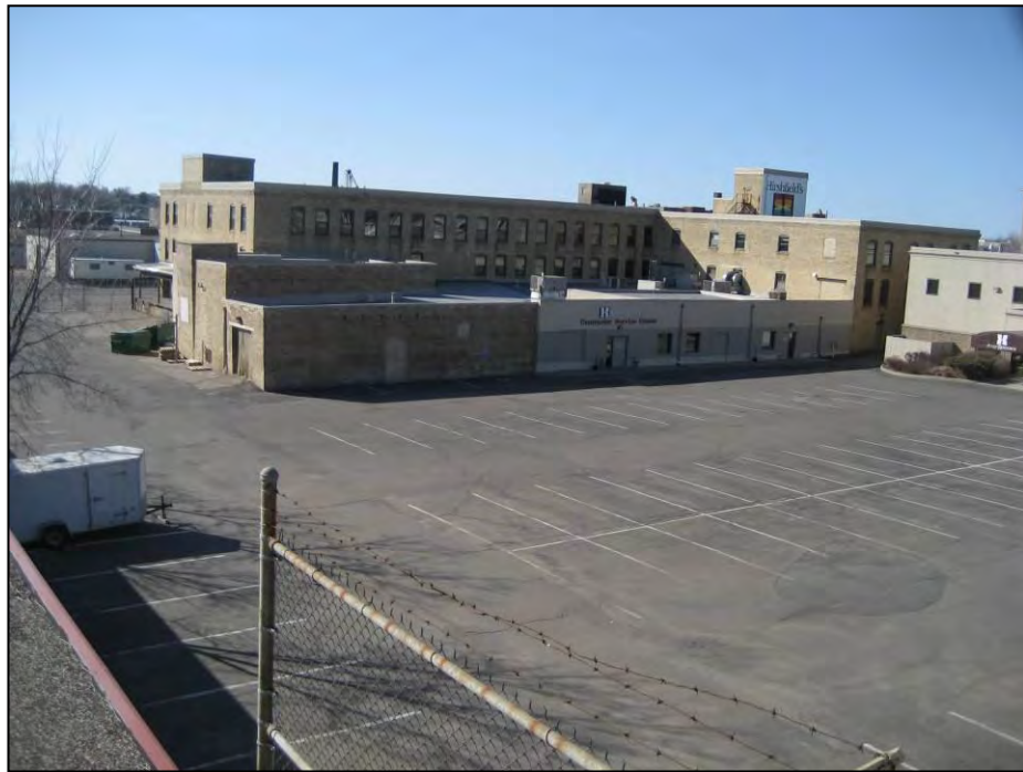
Above: Aldrich facade and rear of building, looking northeast.
