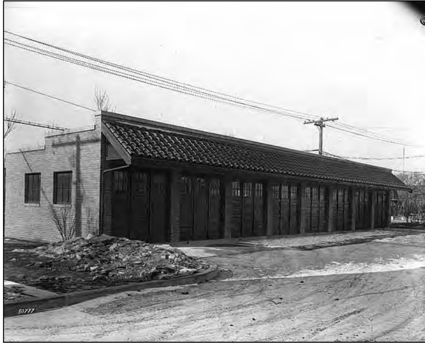
Garage, Hardware Mutual Insurance Company, 1924 Charles Hibbard Photograph—Minnesota Historical Society Collections
