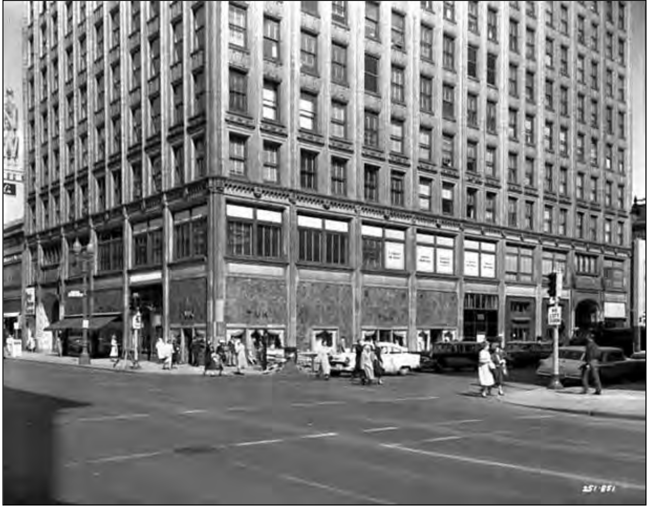
Medical Arts Building, April 23, 1958 Norton and Peel, photographer—Minnesota Historical Society Collections
