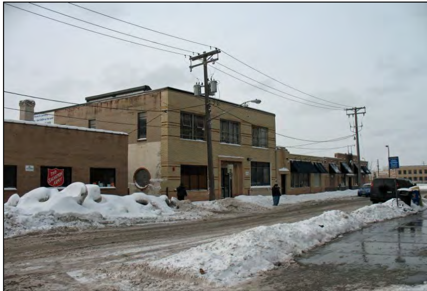
Minneapolis Film Exchange Historic District, view to southwest.
