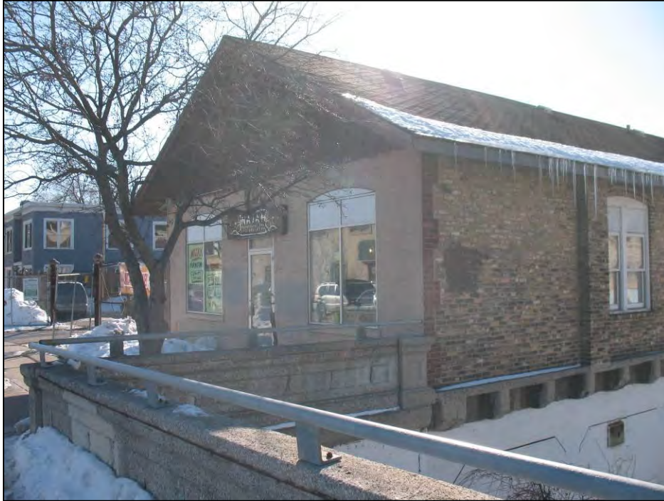
Front (east) facade of the Eighth Ward Warehouse. View to southwest.
