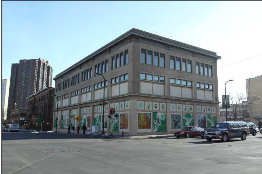
Above: Looking east at the Reno Motor Company (1201 Hennepin Avenue) with Kenosha Flats (1204 Harmon Place) in the background.
