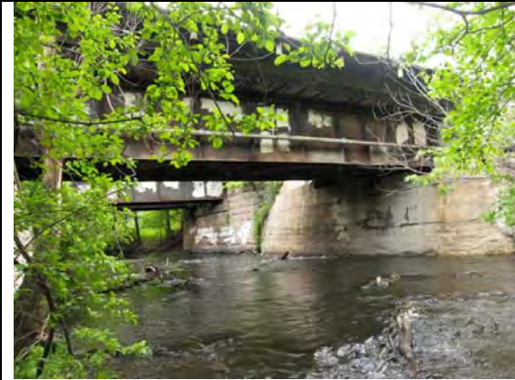
CM&StP Bridge over Minnehaha Creek, facing NE
