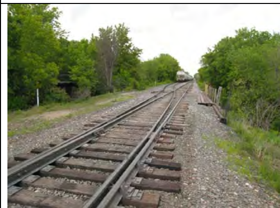
CM&StP Bridge over Minnehaha Creek, facing E
