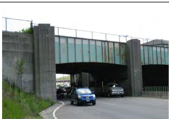
M&StL Bridge over Hwy 100, facing SW
