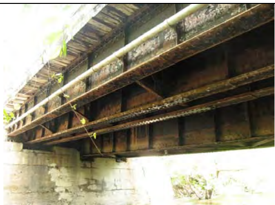
CM&StP Bridge over Minnehaha Creek, facing SE
