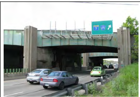
CM&StP Bridge over Hwy 100, facing NW
