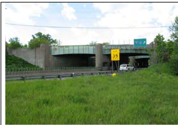
CM&StP Bridge over Hwy 100, facing NW
