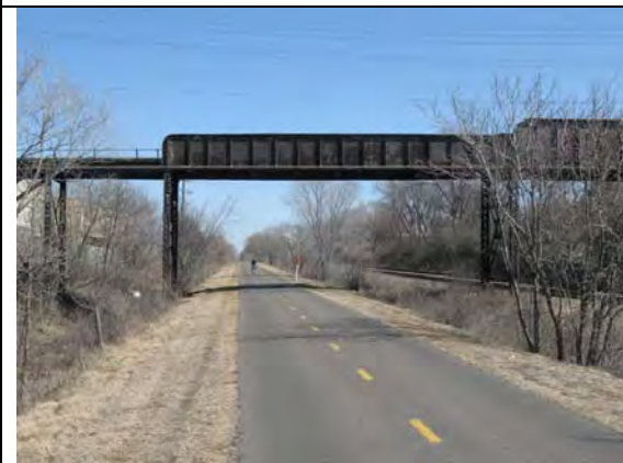
MN&S Bridge, facing E
