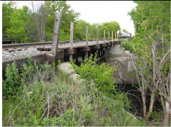
CM&StP Bridge over Minnehaha Creek, facing NE
