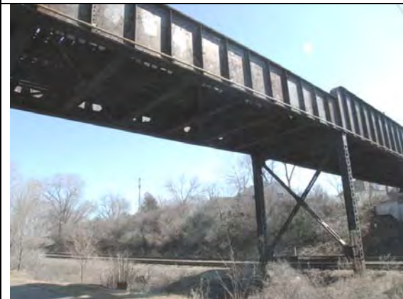
MN&S Bridge, facing SE
