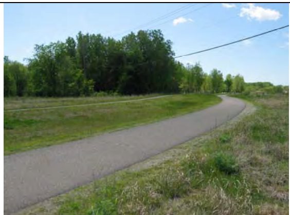
M&StL Corridor in Minneapolis, facing SW
