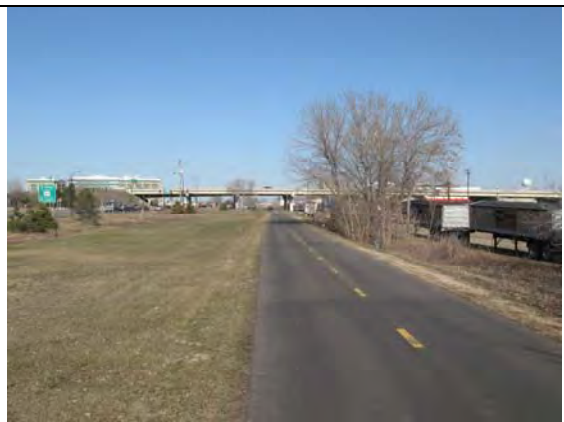
M&StL Corridor in Hopkins, facing NE
