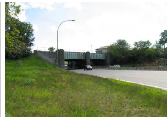
M&StL Bridge over Hwy 100, facing SW
