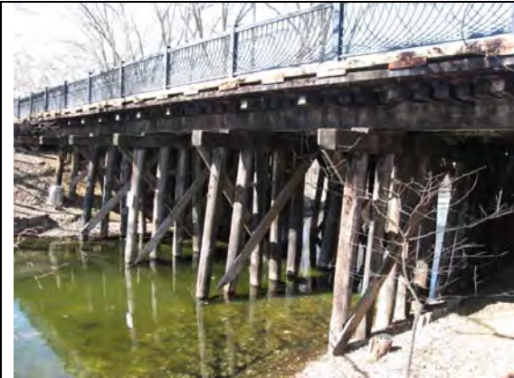
M&StL Bridge over Kenilworth Canal carrying recreational trail, facing SW
