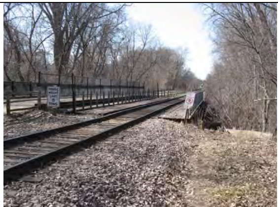
M&StL Bridge over Kenilworth Canal, deck facing W
