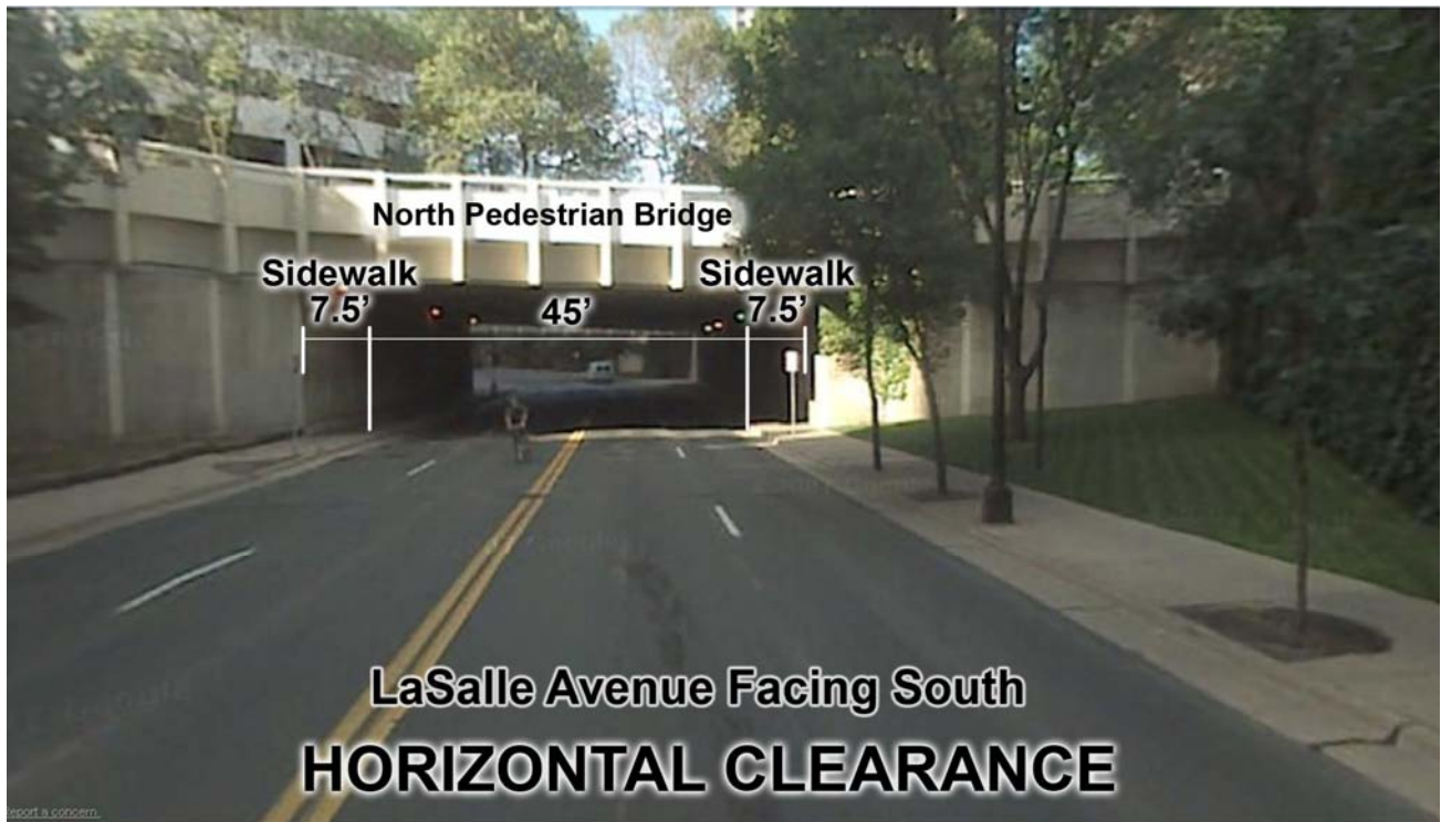
Figure 2: A visual analysis of the tunnel section
