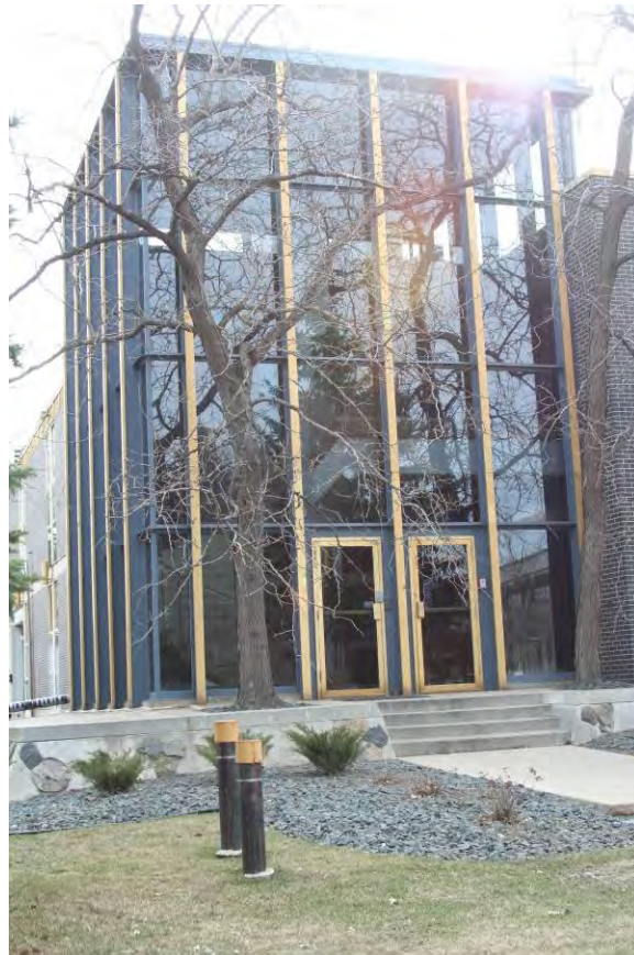
Figure 74. Glass wall corner feature found on the northwest corner of Building #1, added in 1968, view facing southeast.
