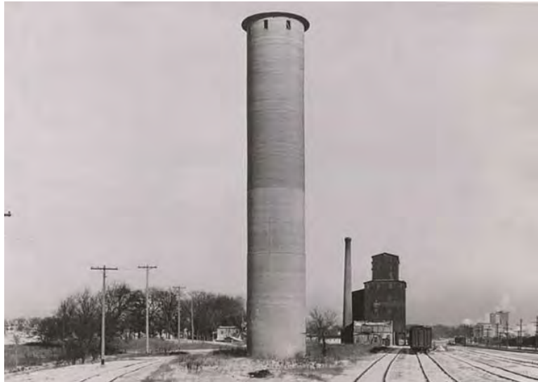
Figure 8. Peavy-Haglin Experimental Concrete Grain Elevator, located along the rail corridor, c.1908 (photo courtesy of the Minnesota Historical Society, Negative 26073).
