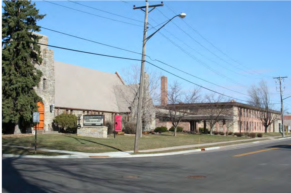
Figure 67. Overview of Union Congregational Church property, view facing northwest.
