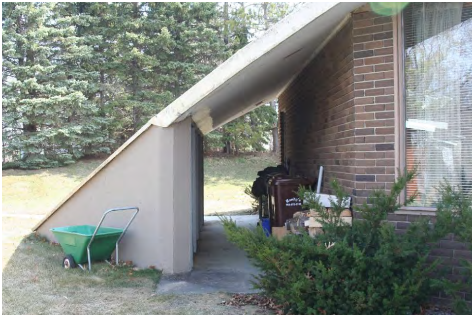
Figure 14. Detail view of the concrete anchors.
