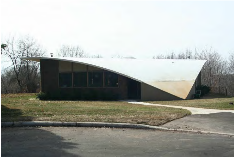
Figure 11. North elevation of the Lang House, view facing south.
