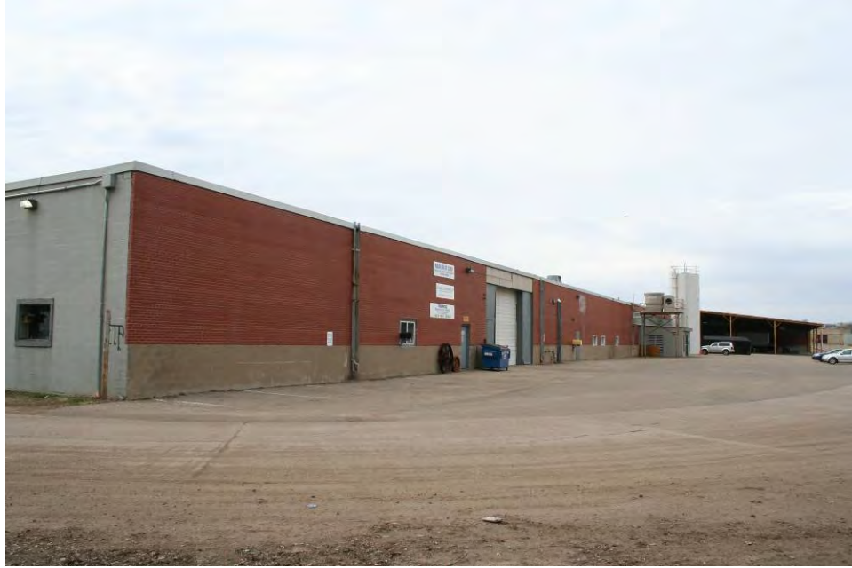
Figure 45. Former Minneapolis Moline building, side (east elevation), view facing north.
