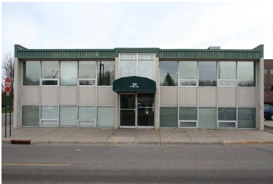
Figure 50. East (primary) facade, view facing west.
