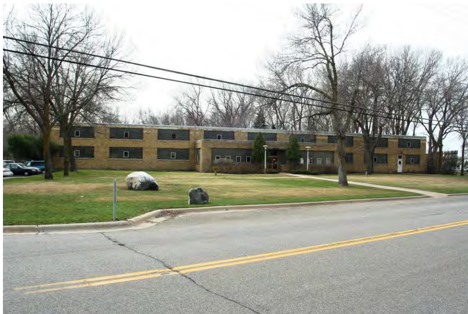
Figure 61. Woodmark Industries Building, view facing southwest.
