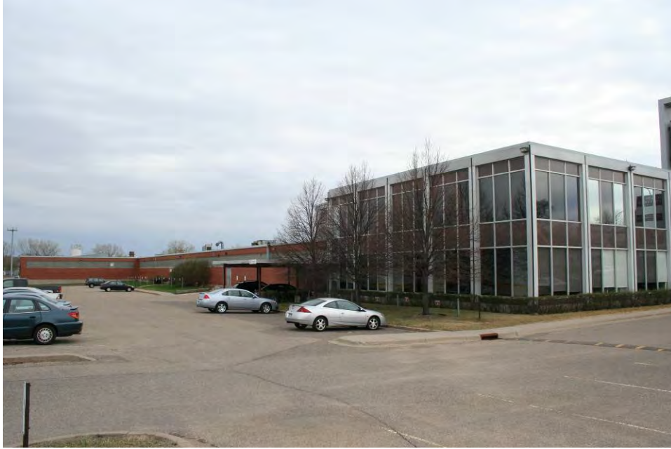
Figure 41. Former Minneapolis Moline building, side (east elevation), view facing southwest.
