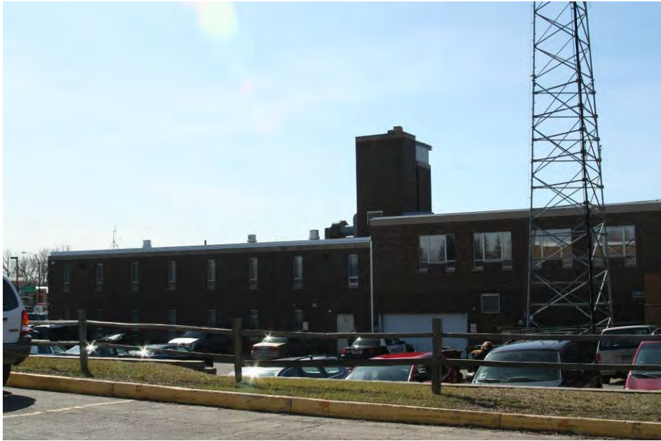
Figure 25. East elevation of Hopkins City Hall, including the hose drying tower, view facing southwest.
