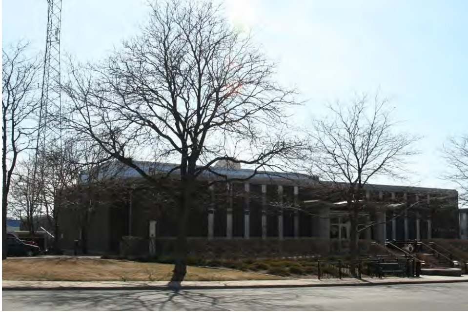
Figure 22. North facade of Hopkins City Hall, view facing southwest.
