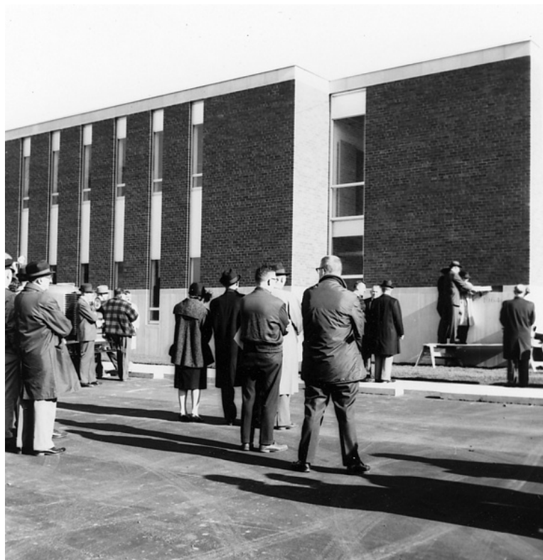
Figure 28. Laying the cornerstone for Hopkins City Hall on the west elevation, November 13, 1964. (Richard Sly, available at www.hopkinsmnhistoricalsociety.org ).
