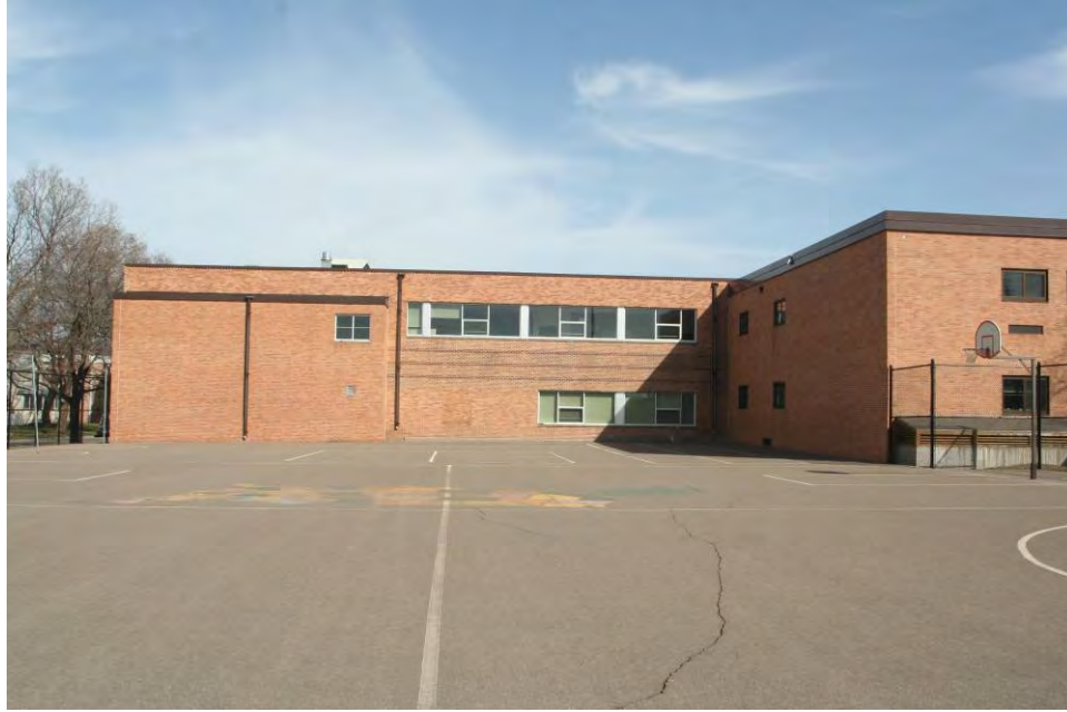
Figure 60. St. Louis Park High School, additions to the rear (north) and side (west) elevation, view facing east.
