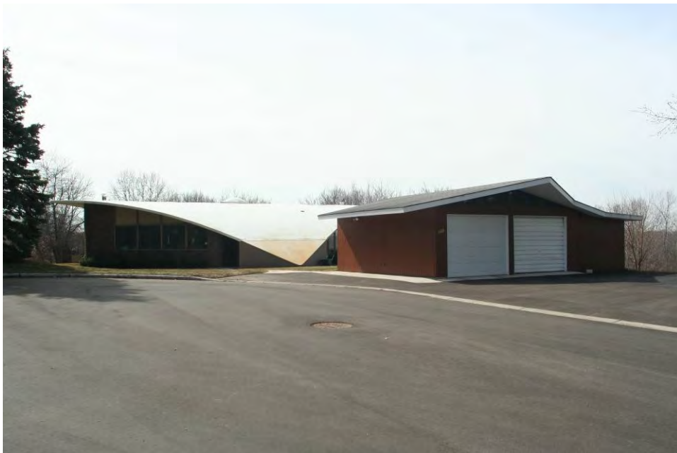
Figure 12. View of the garage and house, view facing southwest.
