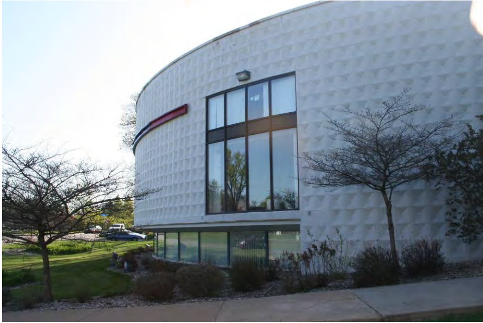
Figure 82. Front portion of the building, view facing southeast.
