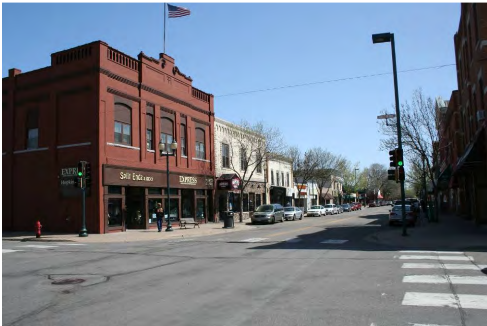
Figure 30. North side of 900 block of Mainstreet, note the IOOF Building on the corner, view facing northeast.
