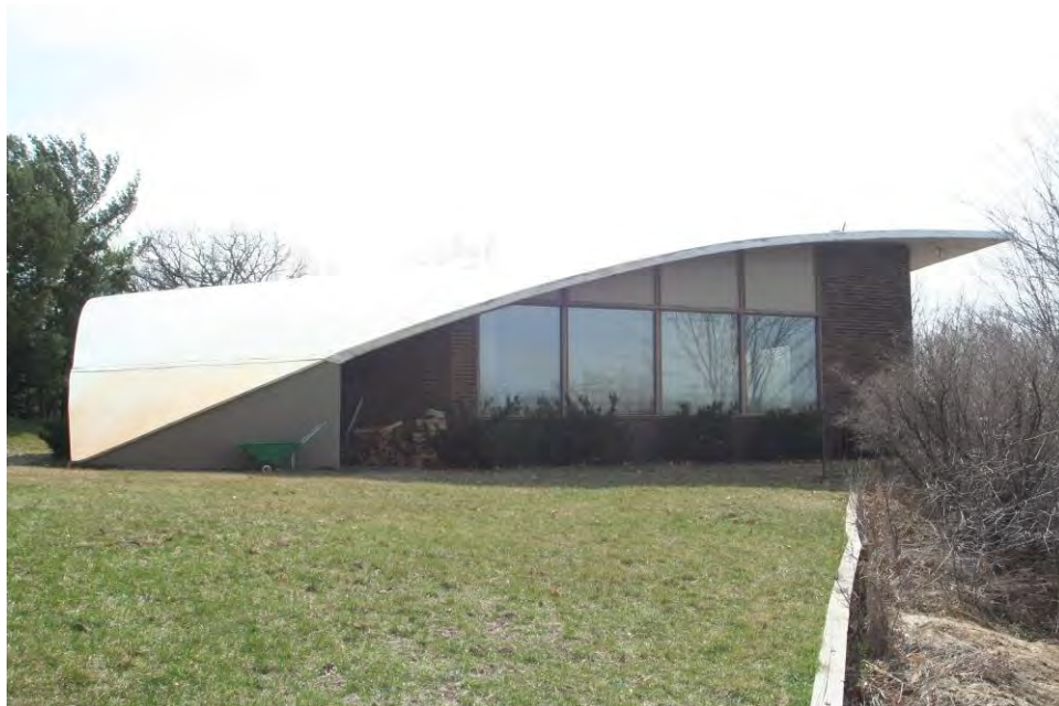
Figure 16. Northwest elevation, view facing southeast.
