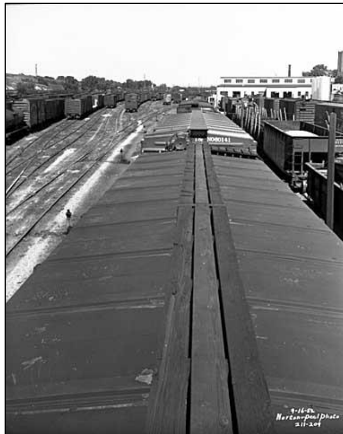
Figure 7. Minneapolis & St. Louis train yards with the Kenwood Water Tower in the distance on the far right (Norton & Peel photograph, Minnesota Historical Society)
