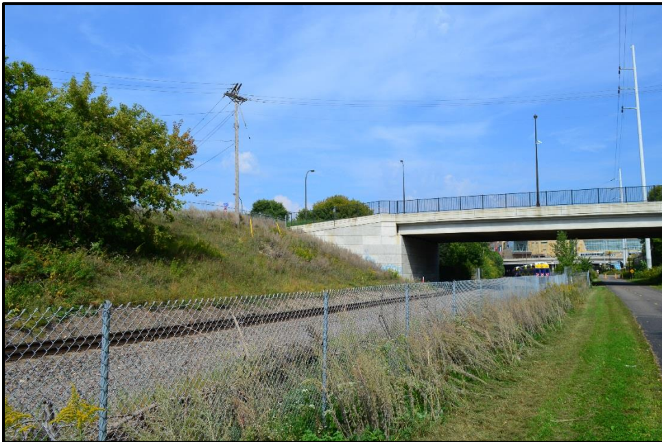
Figure 26. Bluff west of 12th Street on west/northwest side of corridor, August 2017
