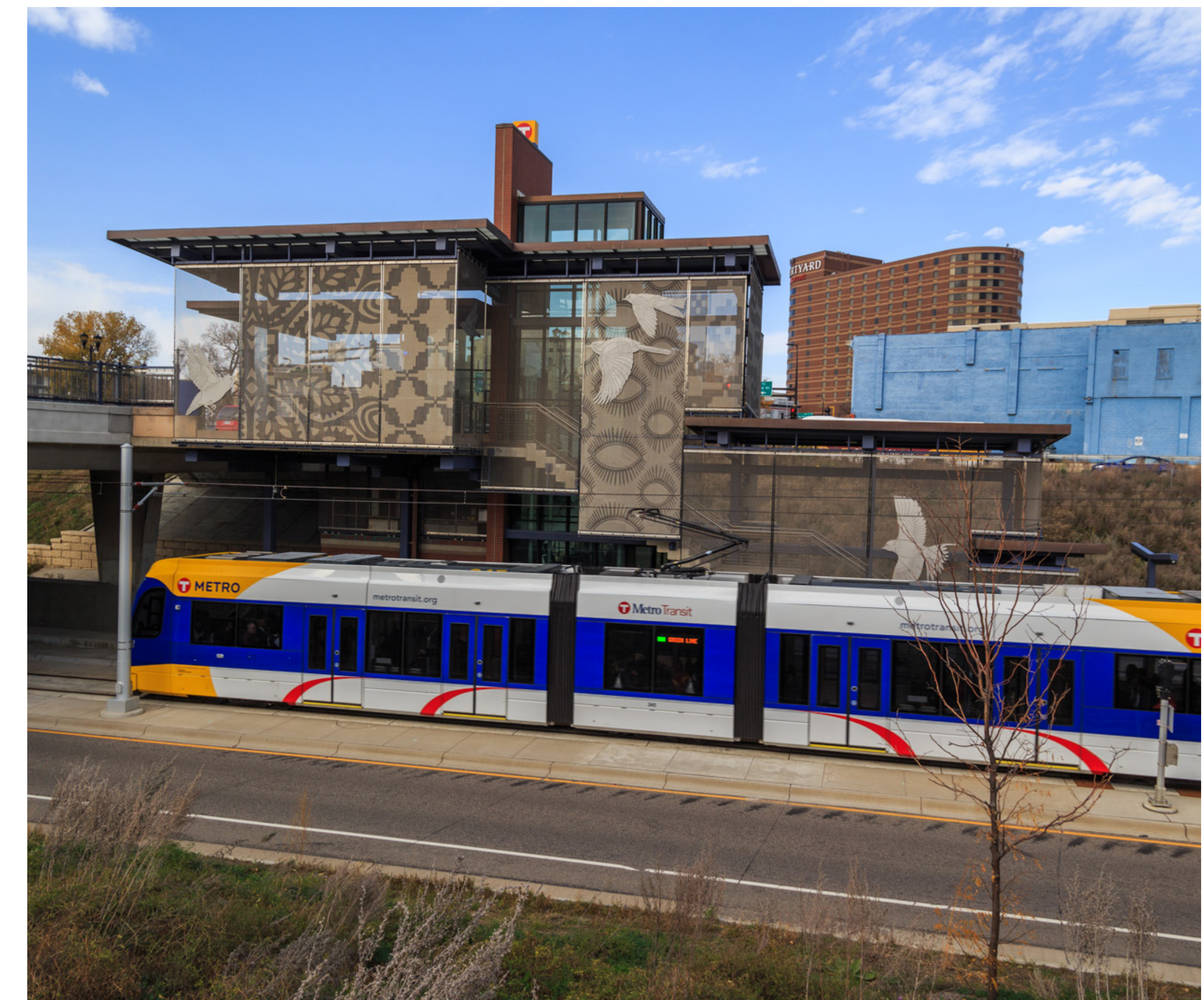
West Bank Station, METRO Green Line
