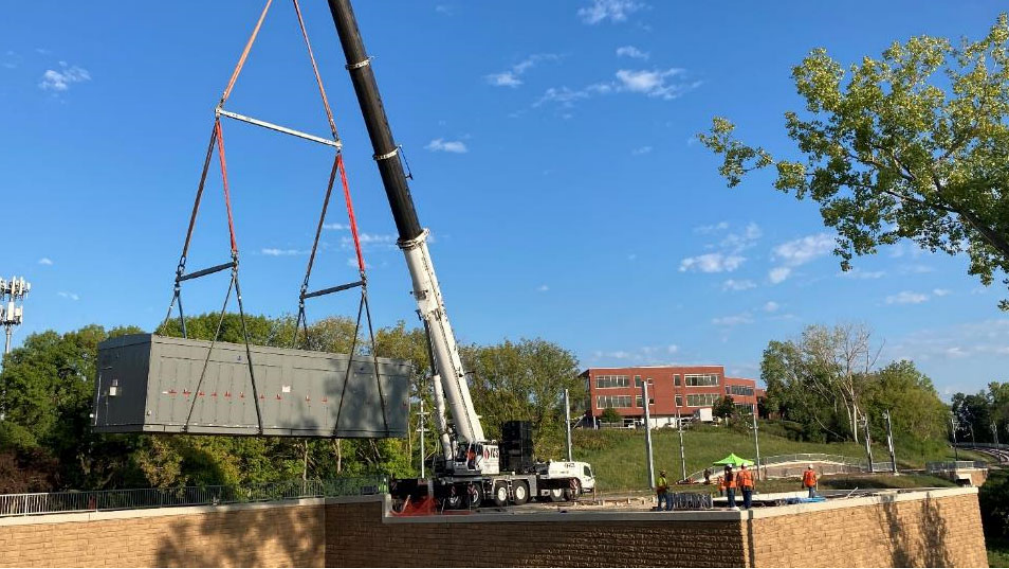
TPSS SW306 Installation in Minnetonka
