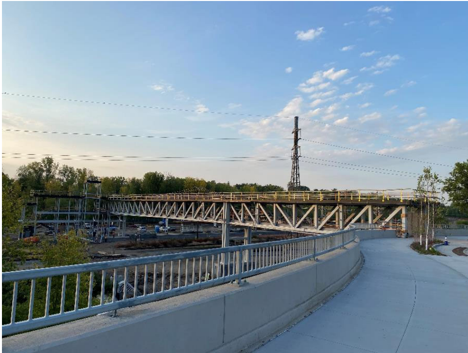
Bryn Mawr Station Pedestrian Bridge
