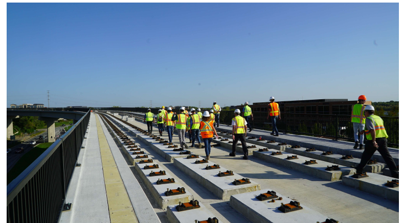
Prairie Center Drive Bridge in Eden Prairie
