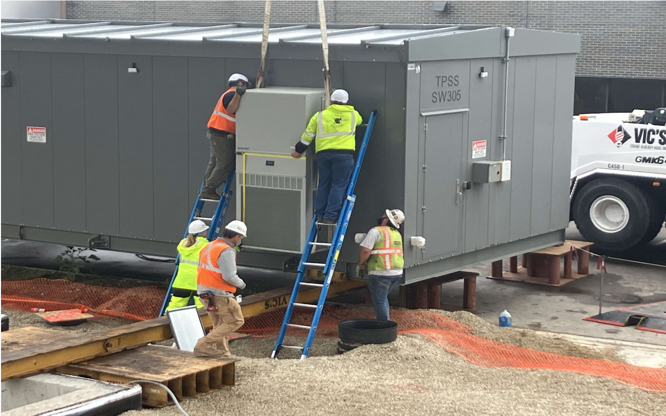
TPSS SW305 Installation in Eden Prairie
