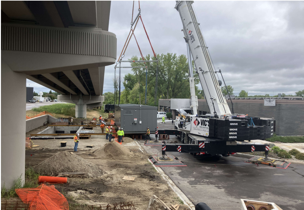
TPSS SW305 Installation in Eden Prairie
