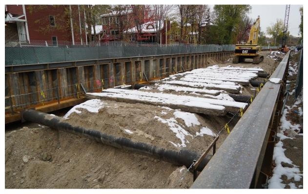
The construction of the Kenilworth tunnel is progressing with a cell-by-cell excavation approach, where 100 feet are excavated at a time. Once sufficient depth is reached, concrete work begins. Specialized equipment is being brought into the corridor to help with excavation.
