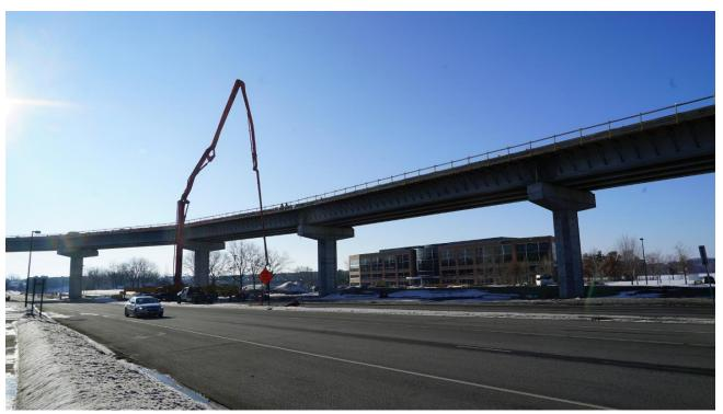
Crews use equipment to place concrete onto the deck of the Prairie Center Drive LRT bridge in Eden Prairie.
