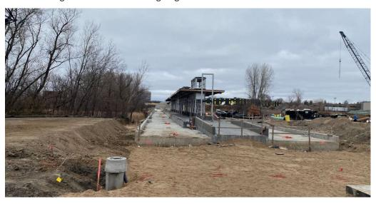
LRT bridge at 212 and Shady Oak: pier work is ongoing, followed by span placement and deck work.
